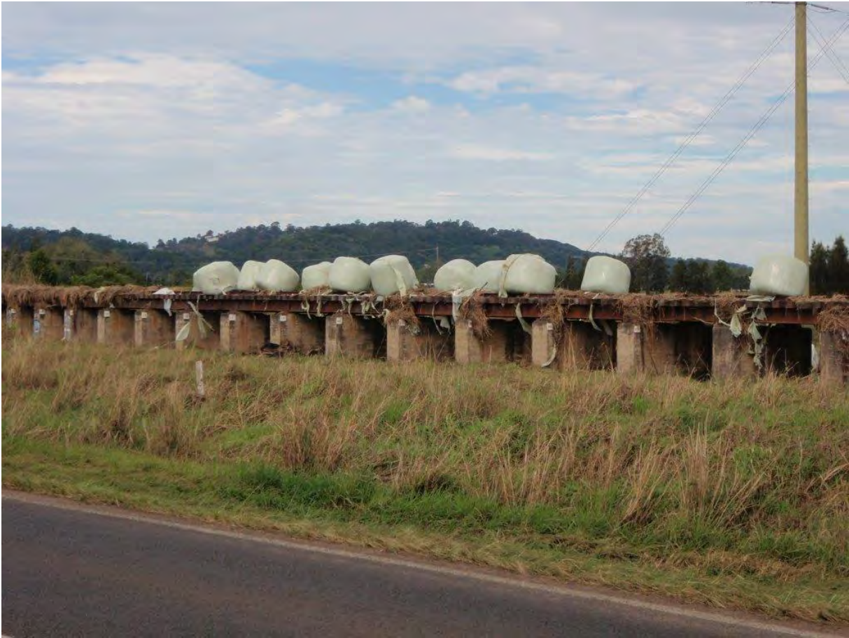
Leycester Creek, Tuncester 23 May 2017, hay bales lifted by the flood onto the railway tracks
