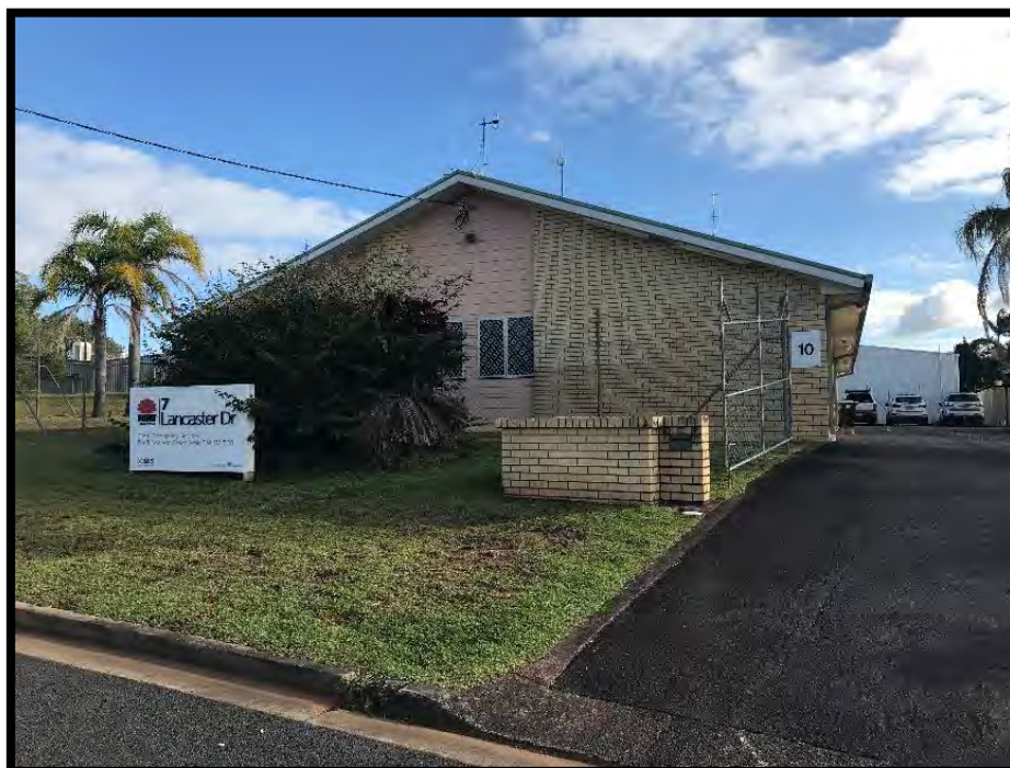
Figure 9: SES Region Headquarters Richmond Tweed
