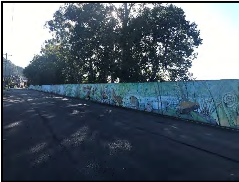
Figure 3: Commercial Road Levee wall (Murwillumbah)
