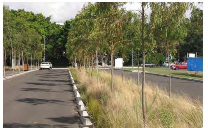
Water sensitive urban design – Integrate water sensitive urban design outcomes into the street, verge and pathway design to increase opportunities for stormwater infiltration and provide additional shade.
