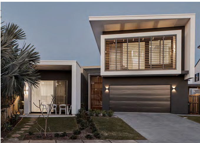
Principle 5: Address the street – Provide a legible front entry with habitable rooms or decks which overlook the street.
