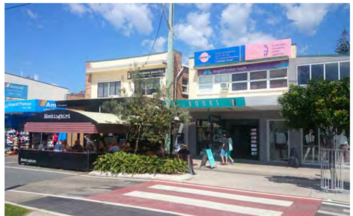
Narrow fronted (fine grain) shops and lower building forms combined with wider footpaths and outdoor dining areas underpin Marine Parades streetscape character.
