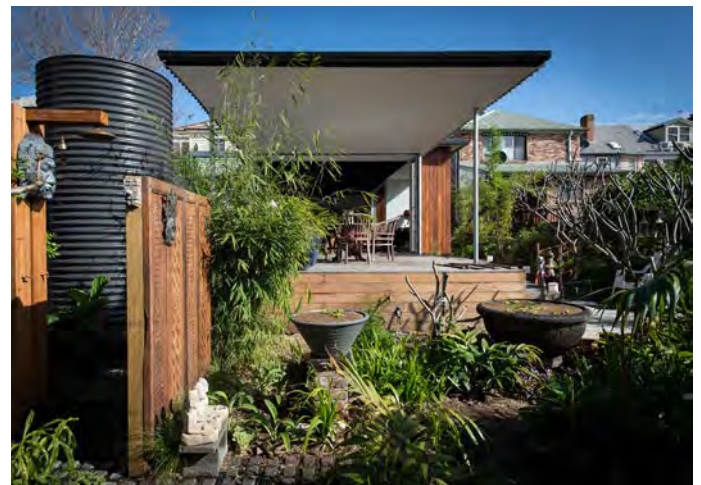
Principle 6: Integrate landscaping – Design yard areas to provide shade, privacy and generous planting areas.
