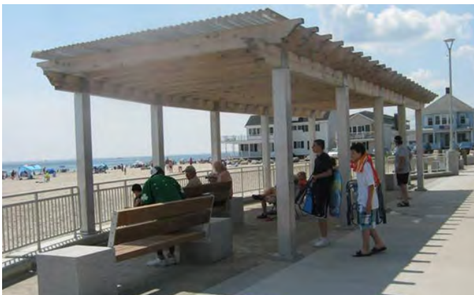
Shade structures within the public domain improves pedestrian and visual amenity.
