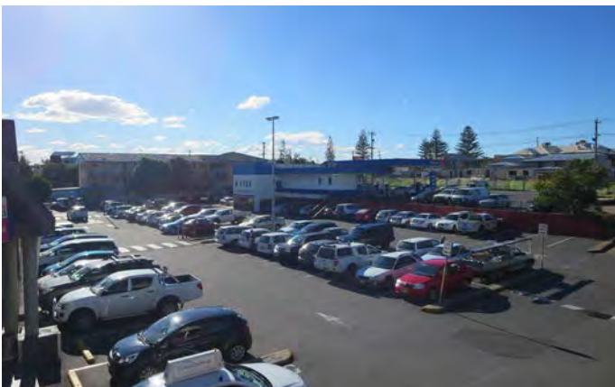
Kingscliff Village Shopping Centre has the opportunity to accommodate a multi-deck and basement car park as part of a future staged redevelopment strategy.
