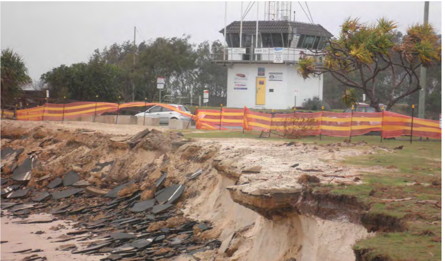
A storm in 2009 caused a significant erosion event along Kingscliff Beach.
