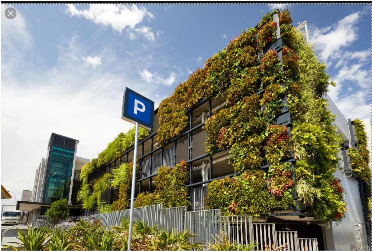
B-Line Commuter Car Park Manly Vale Credits Simon Freeman 2019 C/O Google
