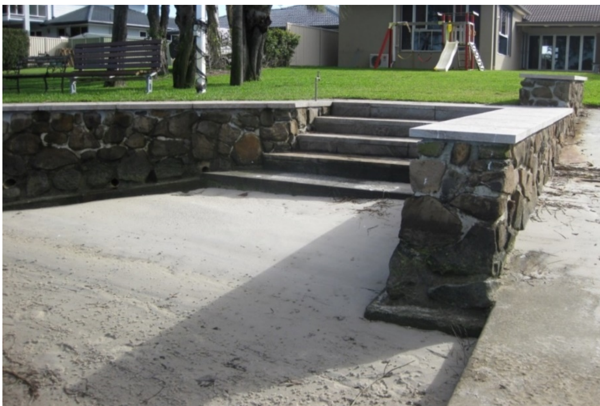
Figure 3: Existing near-vertical rock and concrete retaining wall, stairs and boat ramp adjacent to 20 Wyuna Road.
