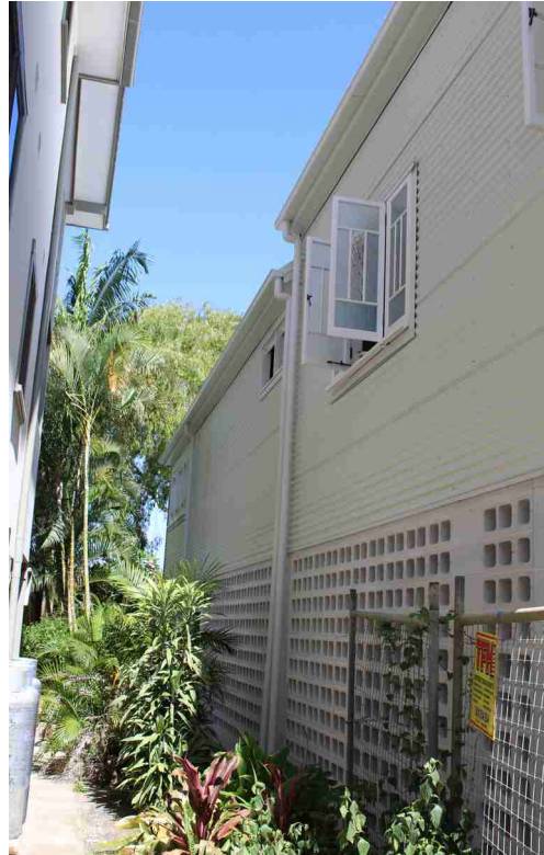
Photograph 5: View from South-East (Between Flats and Dwelling)
