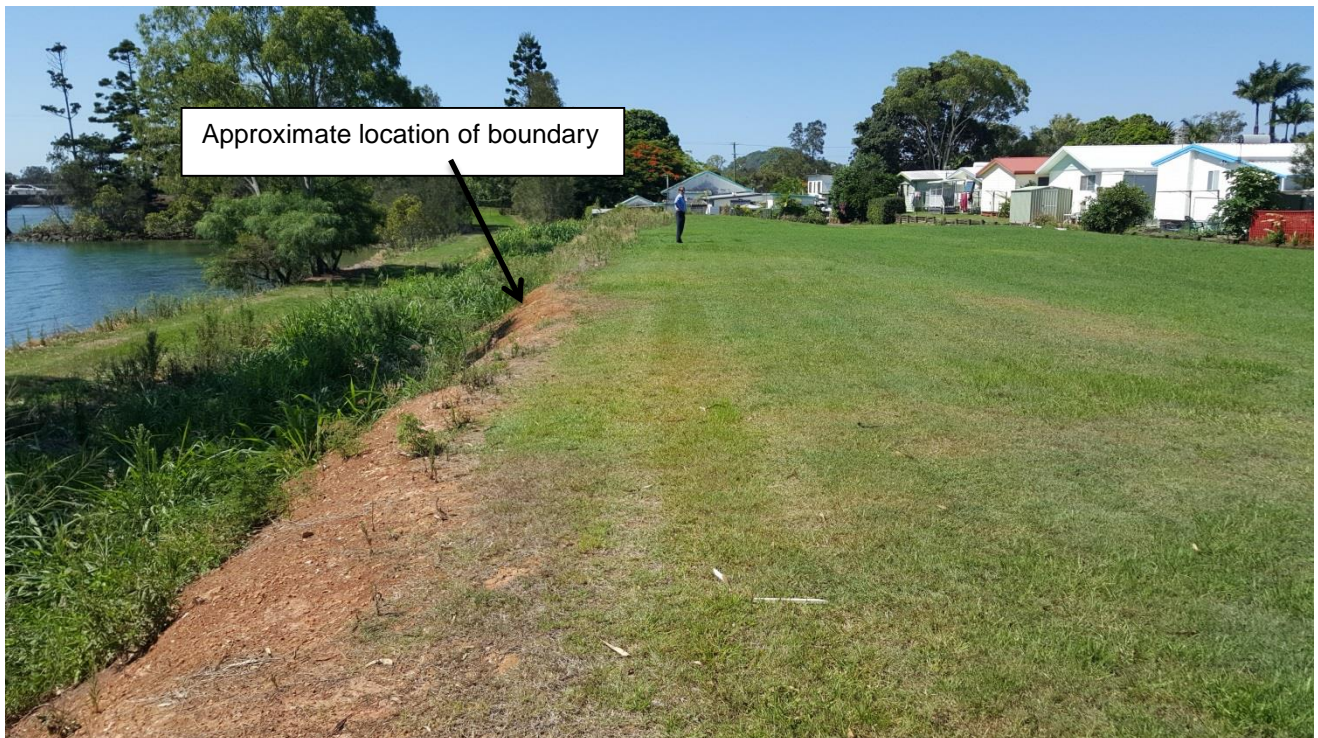
Figure 6: Eastern boundary of site showing depth of fill
