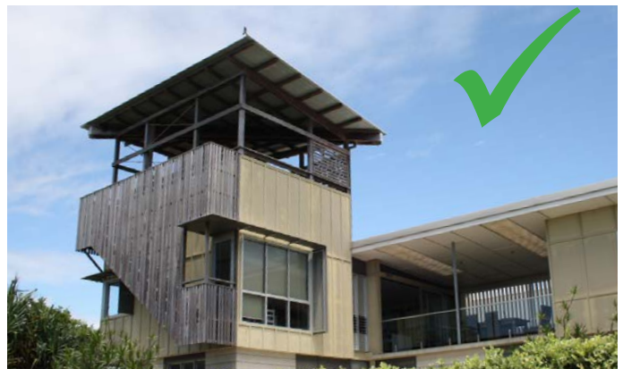
This rooftop terrace has been designed to be compatible with the dwelling by way of form, materials and roof structure and adds architectural interest. A solid balustrade and screening have been included to mitigate potential for overlooking.
