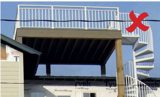
This rooftop terrace fails to be adequately integrated with the dwelling with the structure and stair access being visually dominating. The design does not include any measures to reduce opportunity for overlooking.
