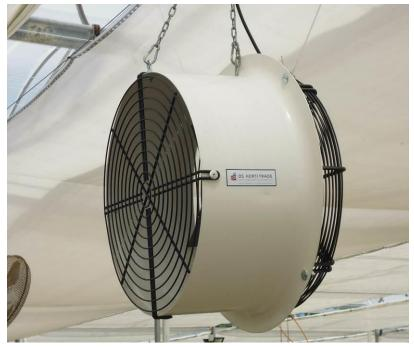
Photograph 1: HAF fans installed in the facility
