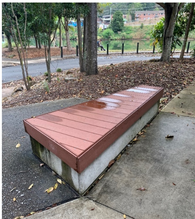
Figure 5: A mixture of composite plastic decking over in-situ concrete in Budd Park designed to be functional and flood proof.
