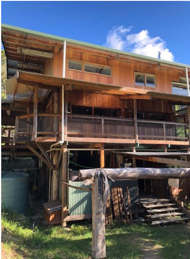
Figure 2 – The already constructed dwelling at No.33 Forest Way.
