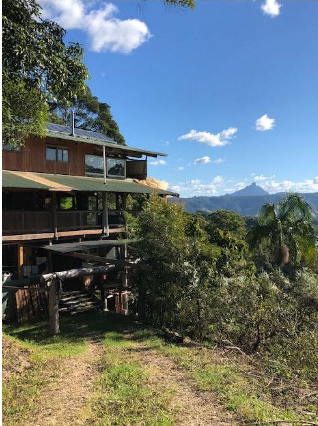
Figure 1 – The already constructed dwelling at No.33 Forest Way.
