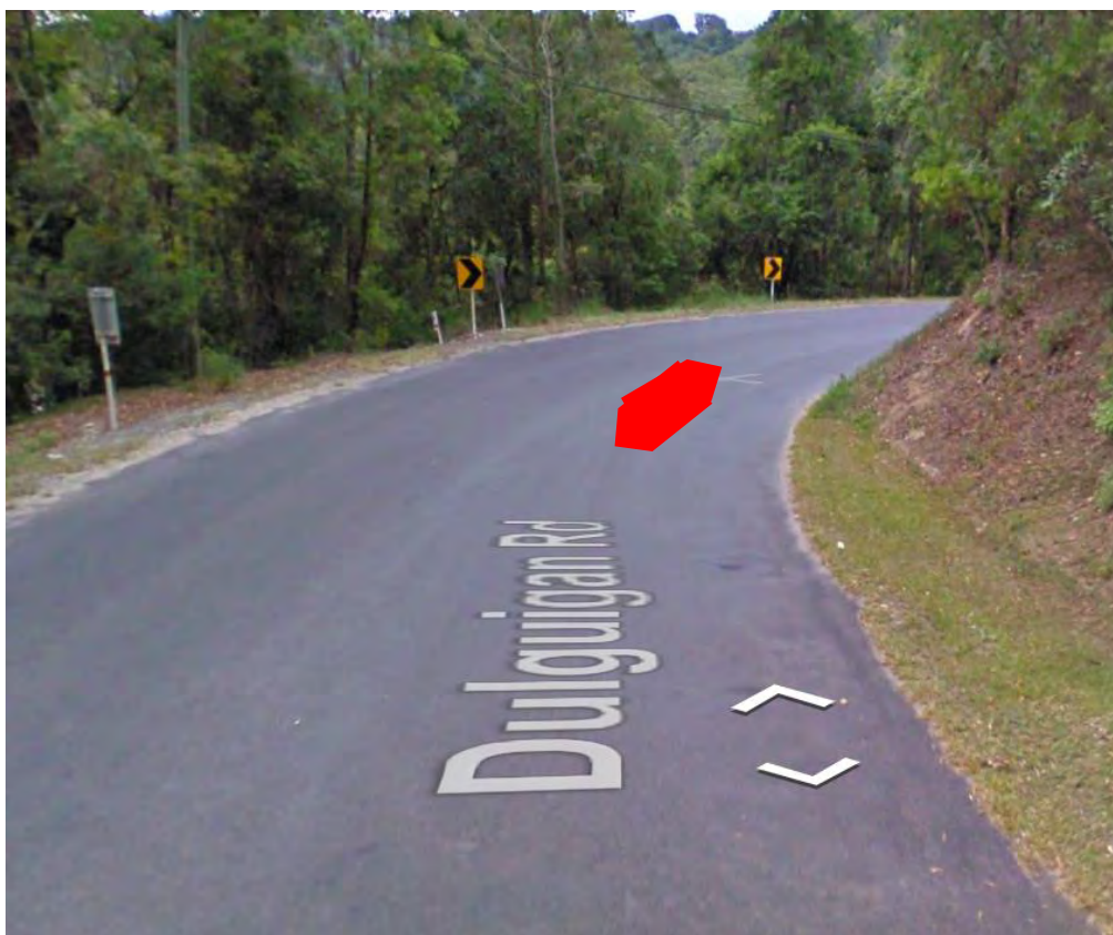
Photo 7.6 Dulguigan Road - looking north
