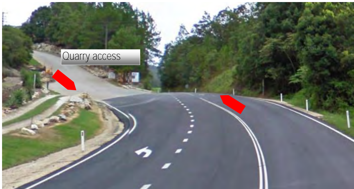
Photo 7.1 Dulguigan Road - looking north-east
