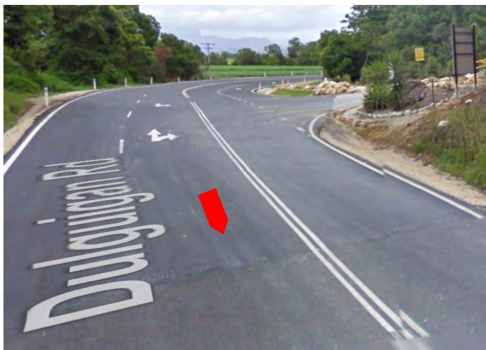
Photo 7.2 Dulguigan Road - looking south-west
