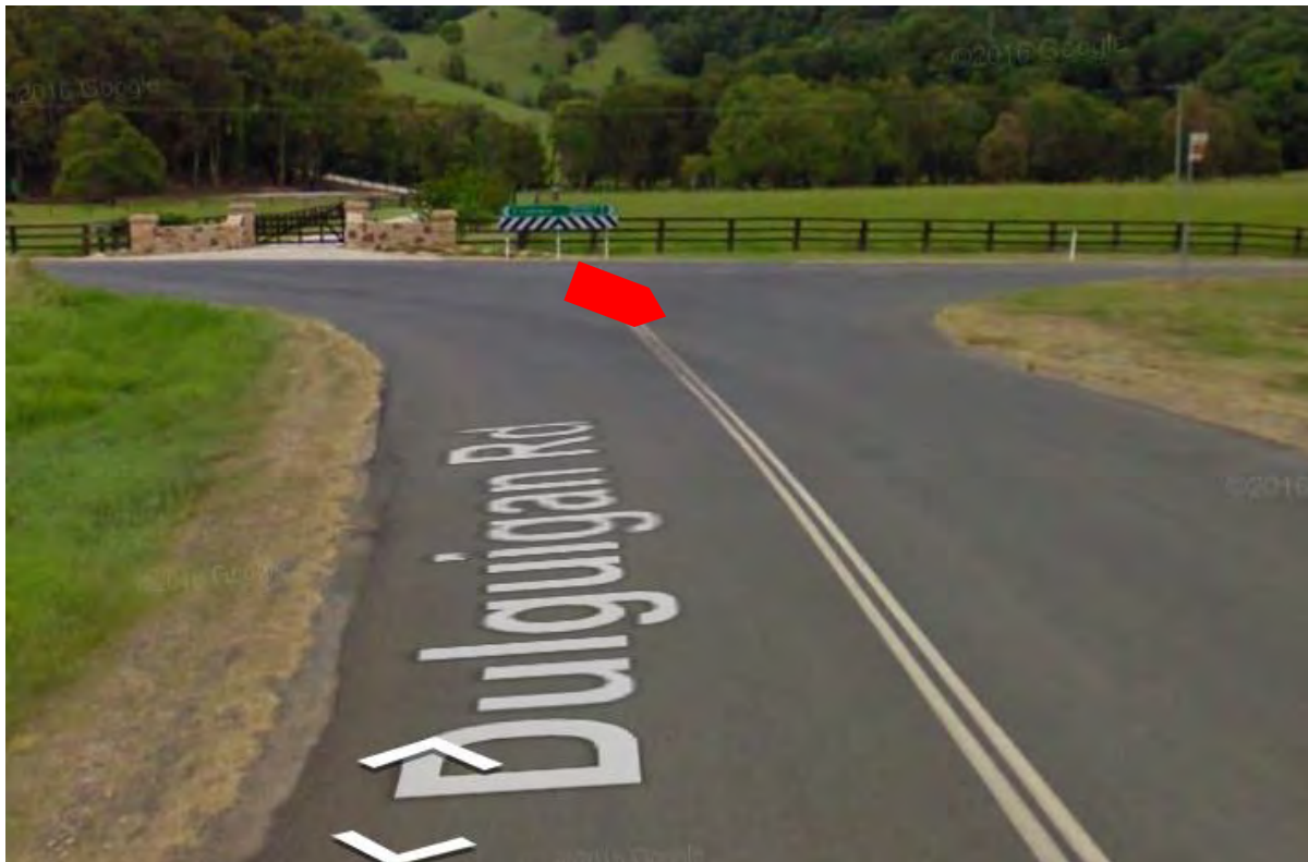
Photo 7.7 Dulguigan Road - looking north-west
