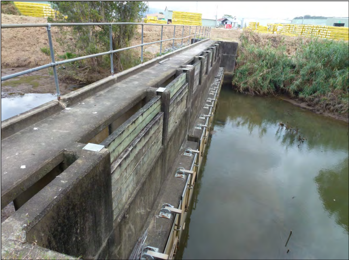
Plate 1 Flood Gate 17L (Condong Creek)
