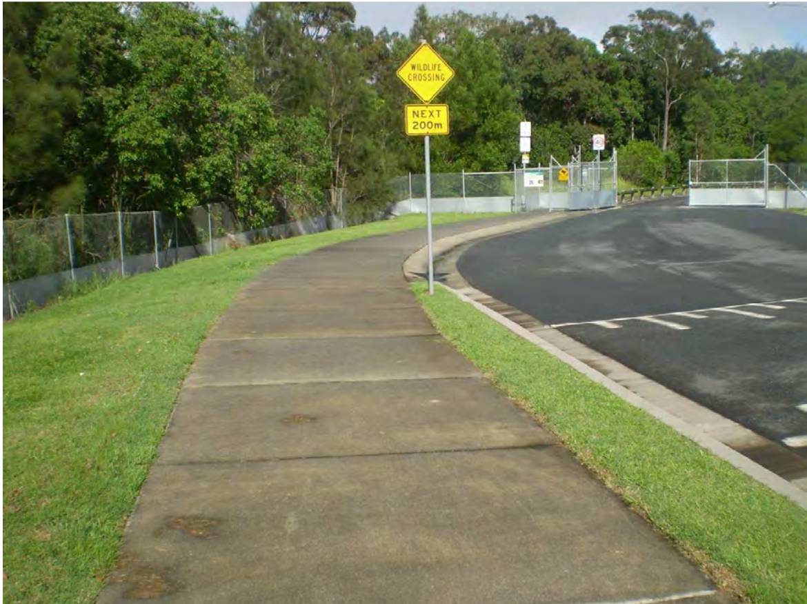
Koala fencing separating subdivision from reserve - cycle way
