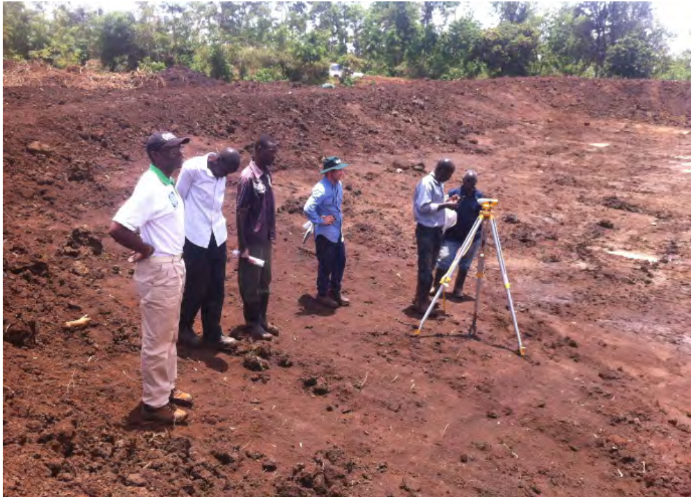
Figure 19: Survey works to determine volume of material excavated.
