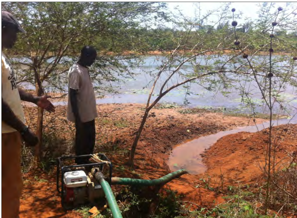
Figure 10: Pumping water at Manyasi Dam.
