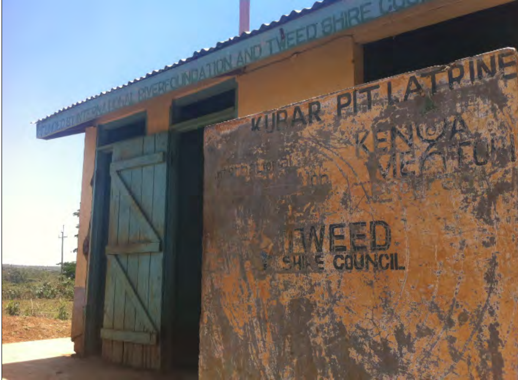
Figure 13: The toilet block at Kubar School located west of Tinga Dam.
