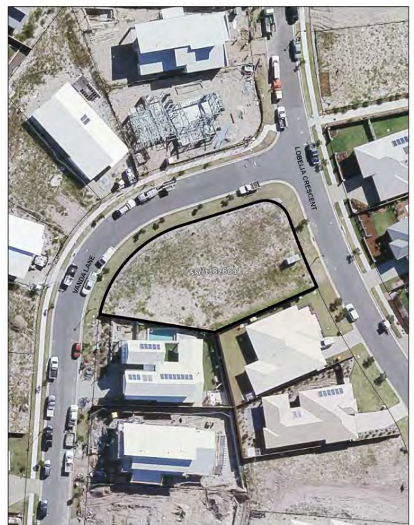
Aerial Photography 2015 Lot 55 DP 1182600 22 Lobelia Crescent, Casuarina (Cnr Vanda Lane) © Land and Property Information (LPI) and Tweed Shire Council Boundaries shown should be considered approximate only
