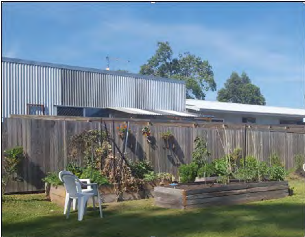
View of the structure from the neighbours property with unapproved awning to the boundary
