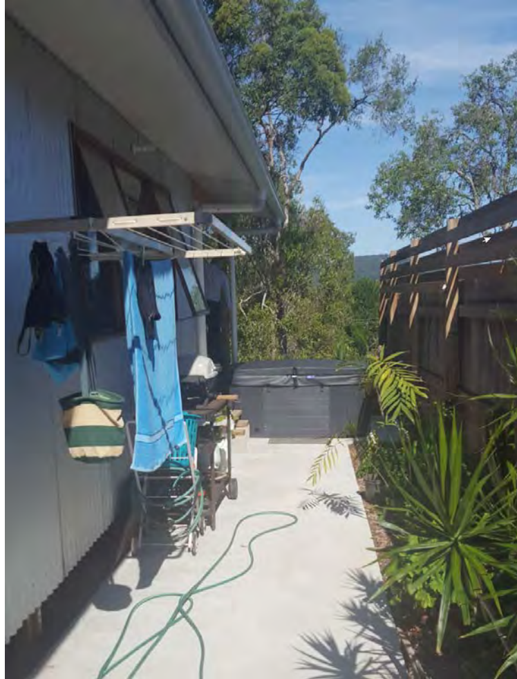
External Spa located on boundary which does not meet the exempt provisions
