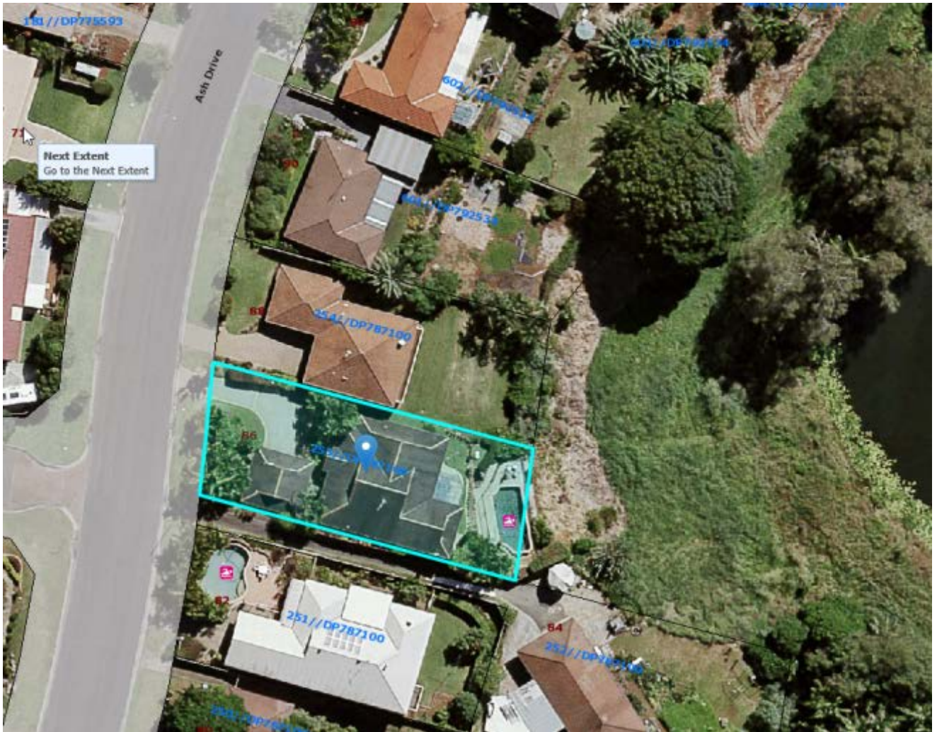
Figure 2 – aerial photo of the subject land, with pool encroaching beyond property boundary
