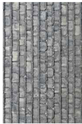
Slate stone roofing
