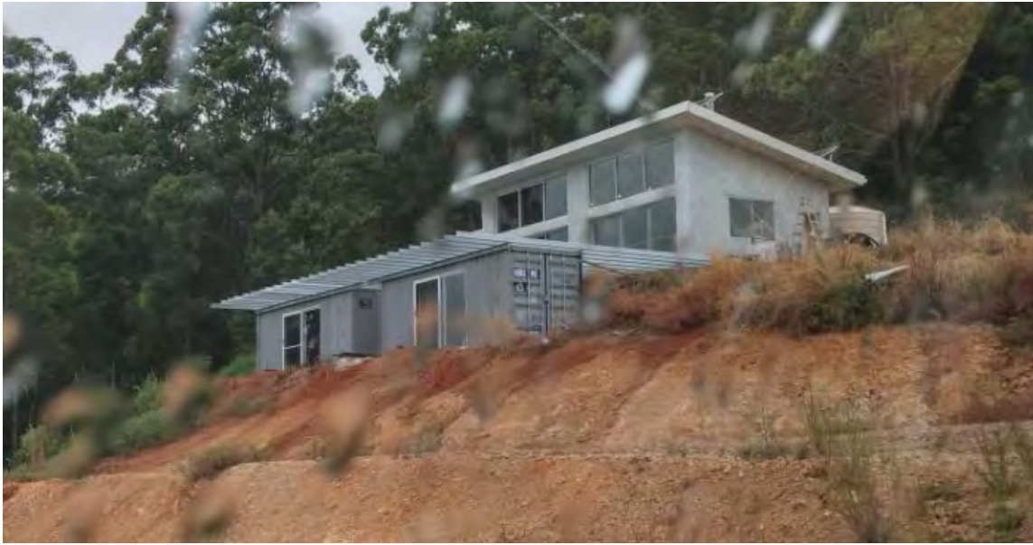
Structure with deck and two shipping containers
