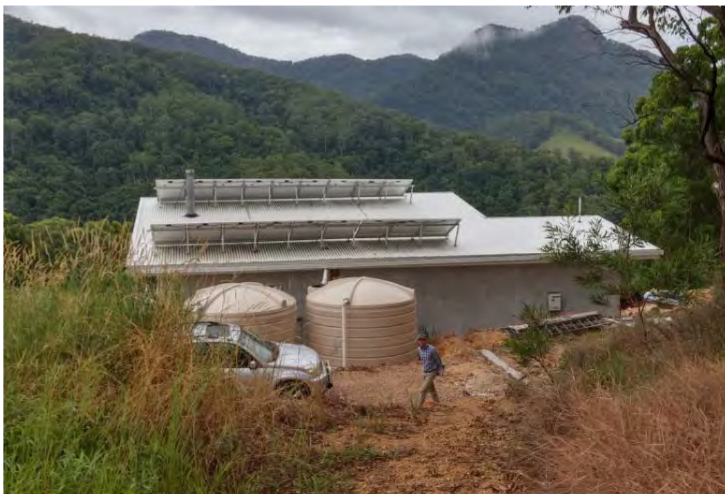
View from rear showing two rainwater tanks
