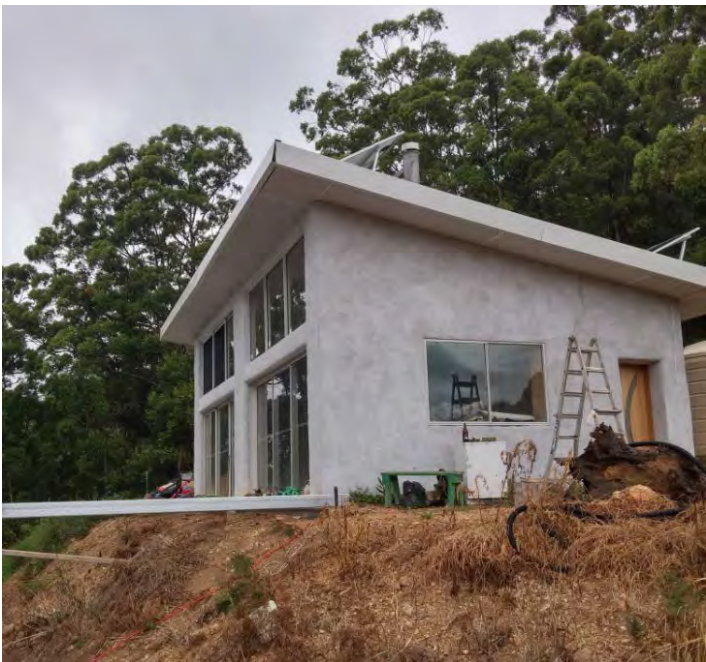
Side view of structure showing front door
