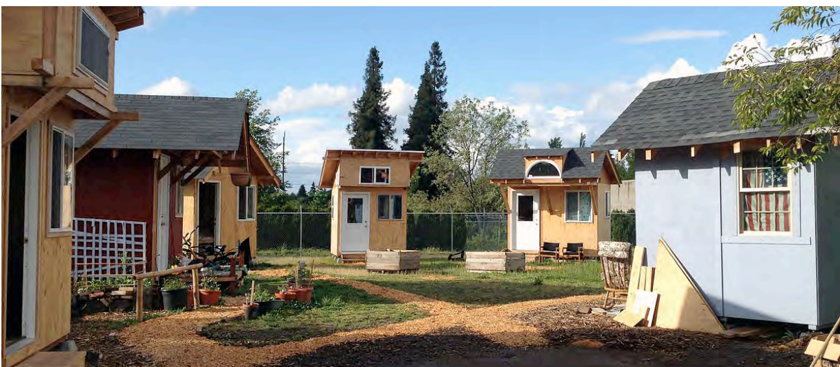
Figure 1 - Example of Tiny Homes Project In Eugene, Oregon, USA
