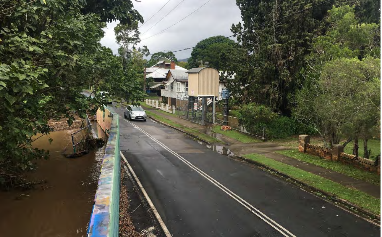
Lavender Creek Pump Station (9:00am on 31 March 2017)
