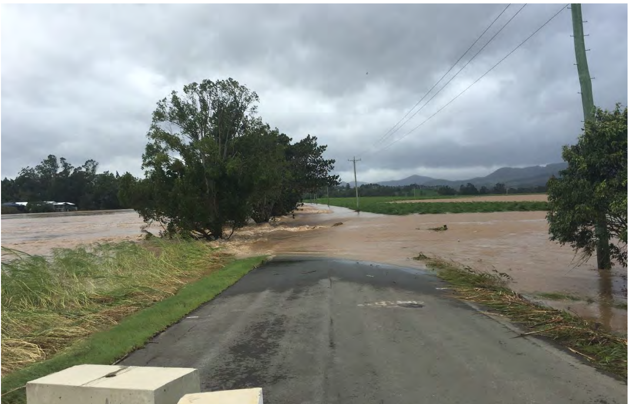
Water spilling across Commercial Road immediately south of levee (9:00am on 31 March 2017)
