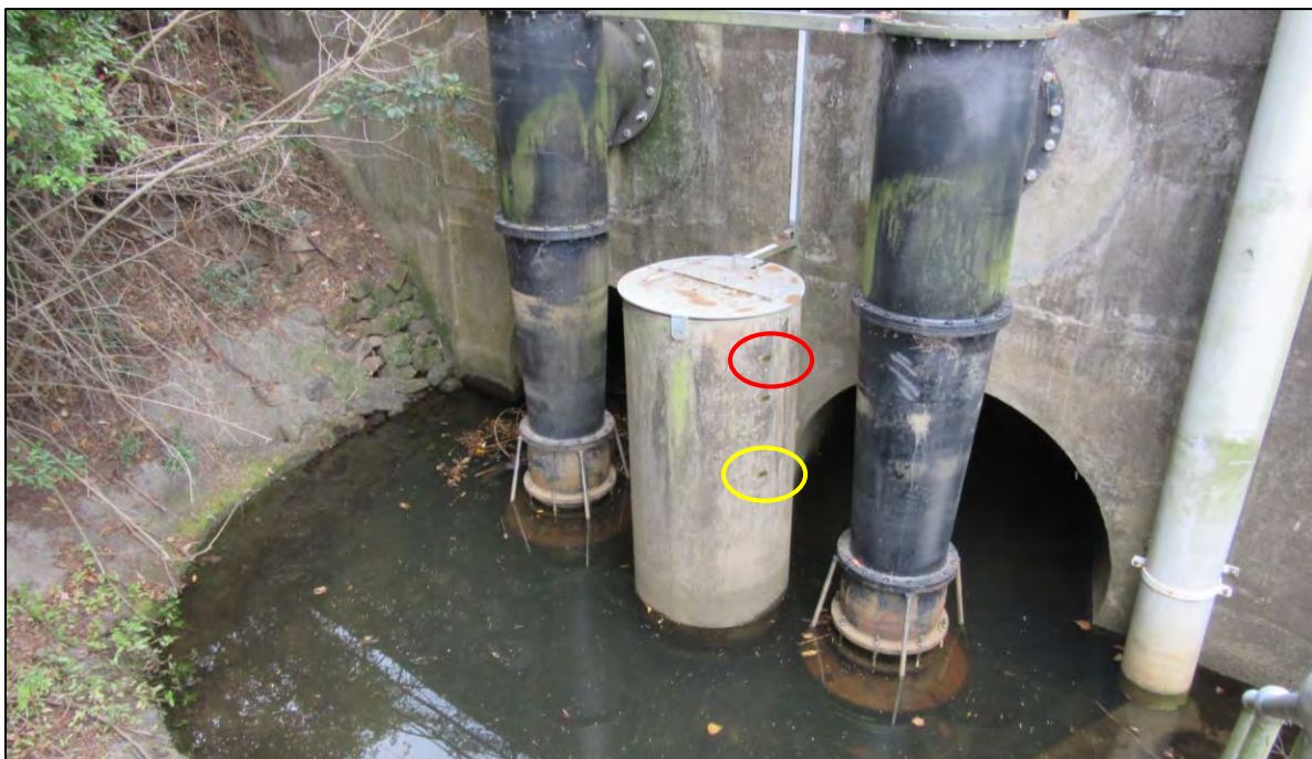
Plate 5 Lavender Creek Flood Pump Station 1 showing vertical intake structures (black vertical structures) and water level sensor (concrete chamber between the black intakes)
