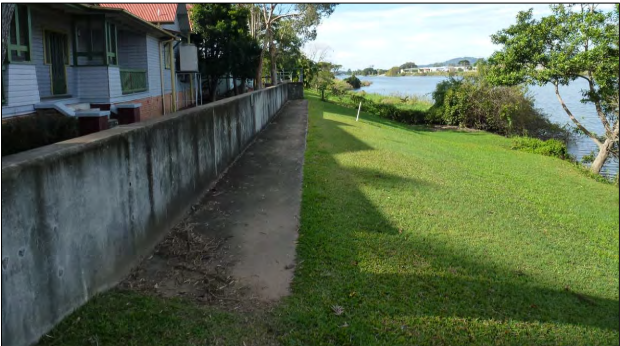
Plate 3 View looking north-east along concrete wall section of the East Murwillumbah levee
