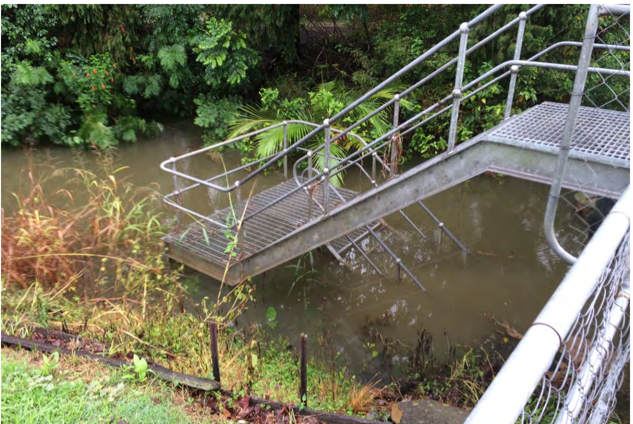
Upstream of Lavender Creek Pump Station
