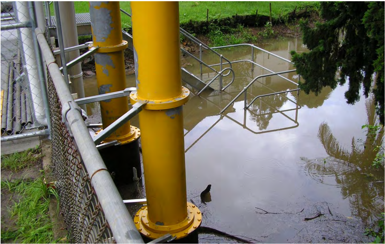
Upstream of Lavender Creek Pump Station
