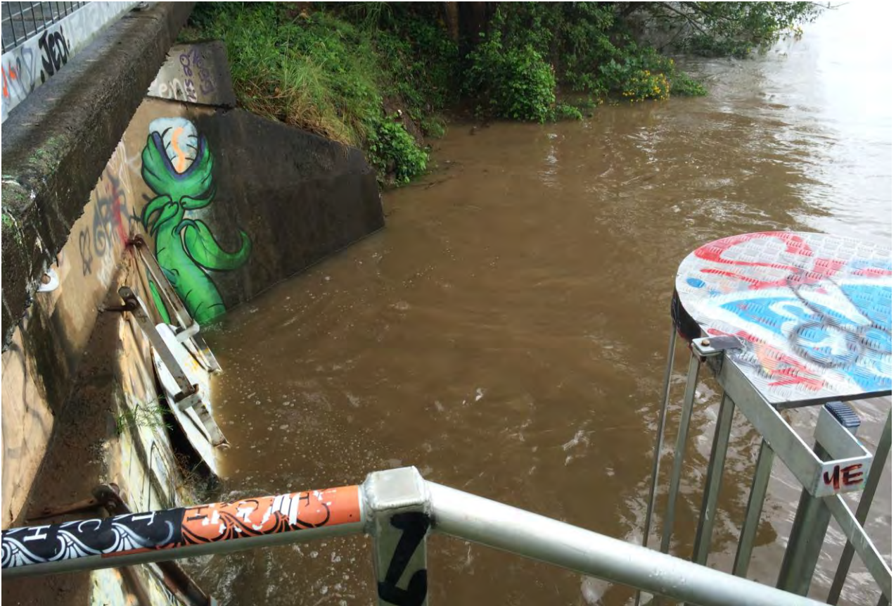
Elevated Tweed River Water Level at Lavender Creek Outlet
