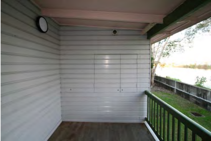
Photograph 73 Kitchen servery to the Southern verandah from early room modified for kitchen
