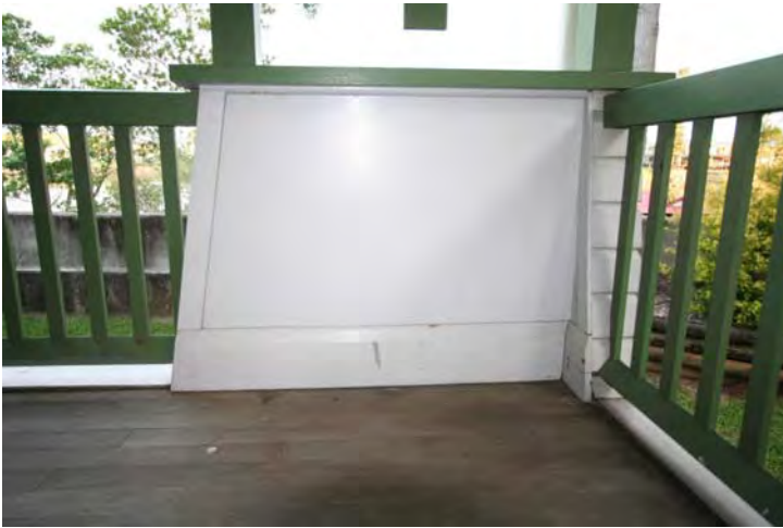
Photograph 68 Verandah detail showing the sheet clad piers
