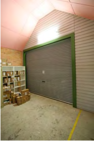
Photograph 138 Loading dock area
