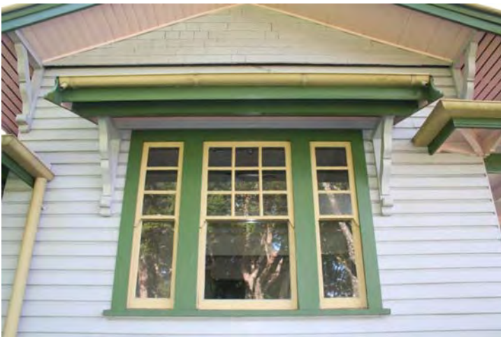
Photograph 33 Original fabric and details – exceptional significance
