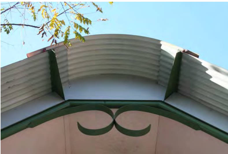
Photograph 42 The extension: Fabric and details – Moderate significance
