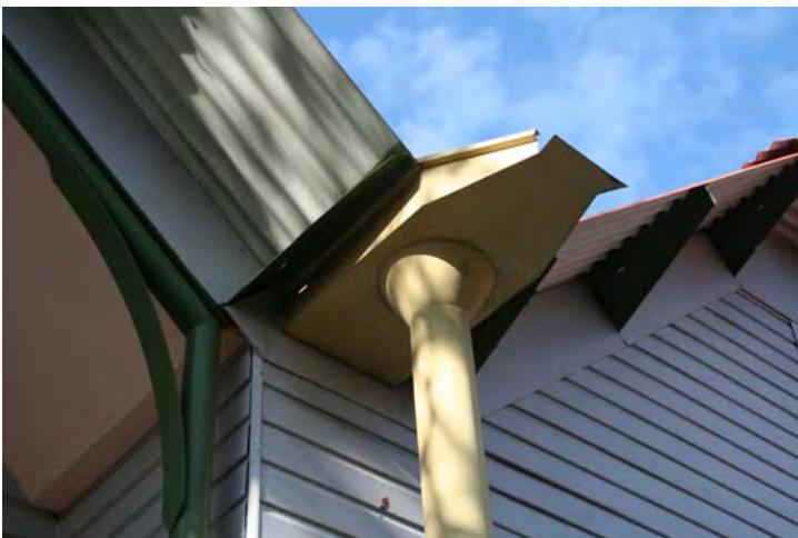
Photograph 41 The extension: Fabric and details – Moderate significance
