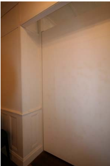
Photograph 6 Little level of significance for removed internal walls
