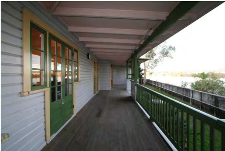
Photograph 69 View East of the Southern verandah, western end
