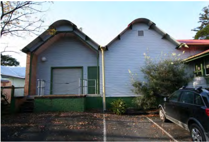
Photograph 65 The sensitive 1988 extension – North eastern corner
