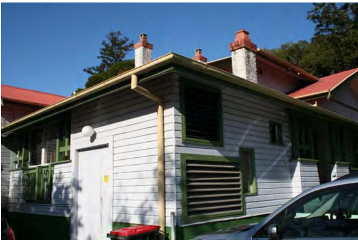
Photograph 23 Former laundry – Modified and Moderate significance
