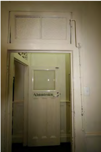
Photograph 104 Original door and toplight with hardware
