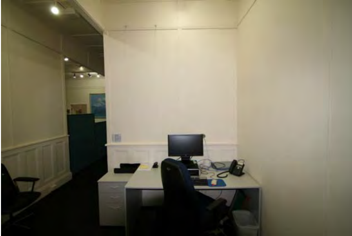
Photograph 117 Retained bulkheads define the former central passage of the residence. Note partition in plasterboard without dado panels
