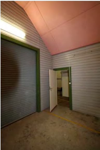
Photograph 139 Enclosed loading dock
