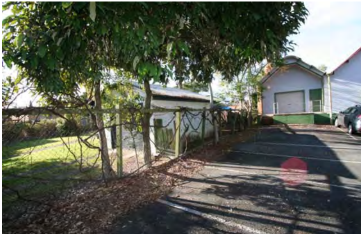
Photograph 44 The extension: Fabric and details and car park setting – Moderate significance
