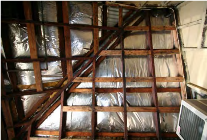
Photograph 11 Modified store-room roof – Moderate significance
