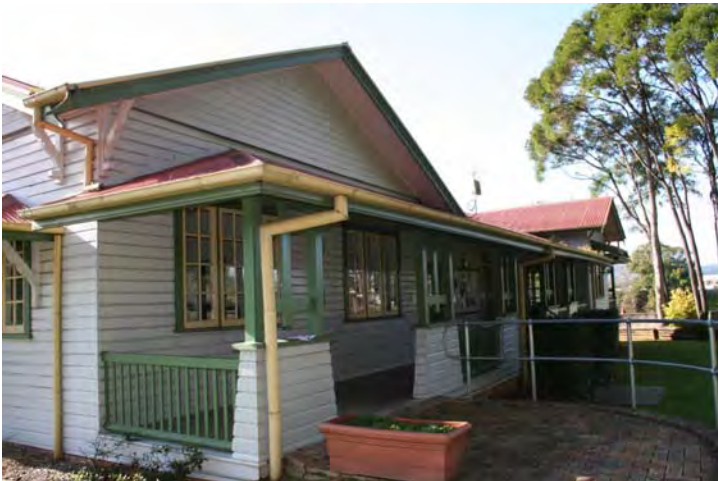
Photograph 26 Front verandah – Modified for ramp and High significance
