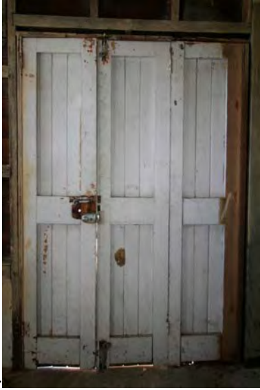
Photograph 10 Original doors – High level of significance
