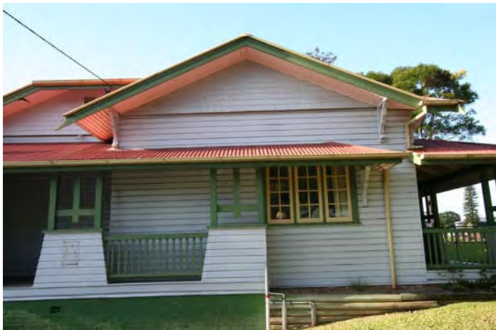
Photograph 63 Exceptional significant and exposed conduit and cables
