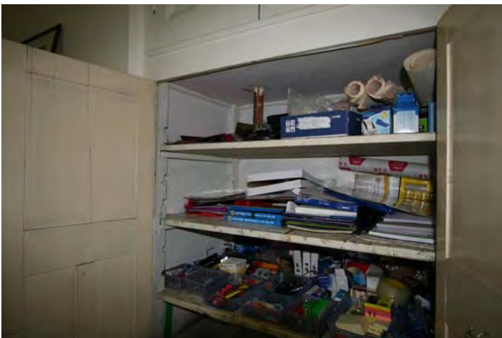
Photograph 90 Exceptional built in cupboard
