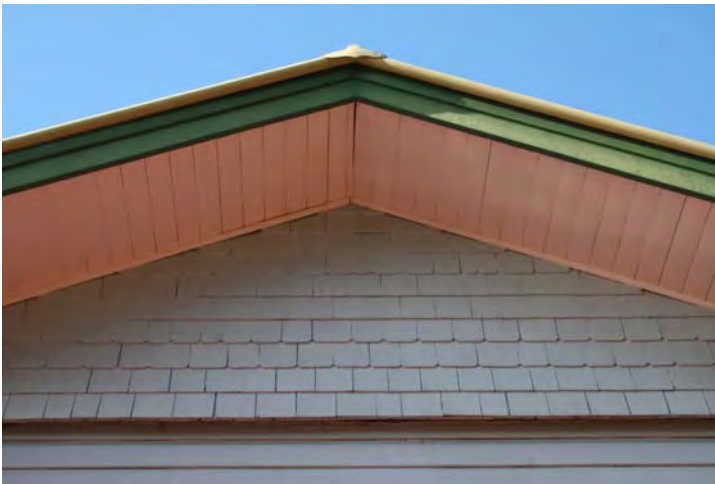
Photograph 38 Original fabric and details – Exceptional significance
