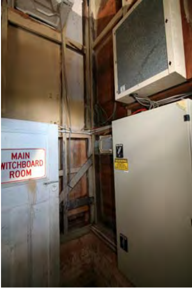
Photograph 15 Former laundry – modified and High significance
