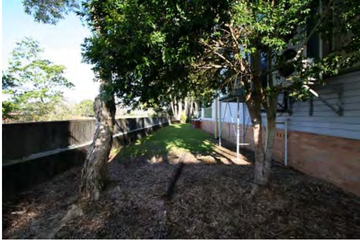
Photograph 61 Setting looking west across the building frontage and AC installation - Intrusive
