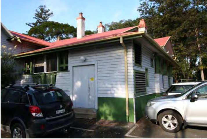
Photograph 64 The Laundry enclosure
