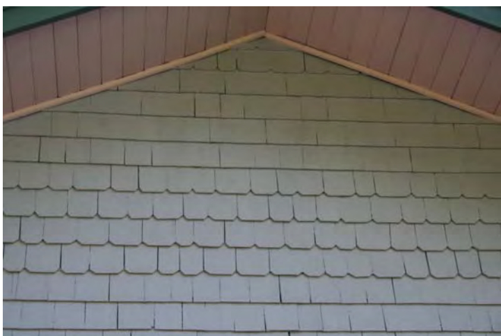
Photograph 36 Original fabric and details – Exceptional significance
