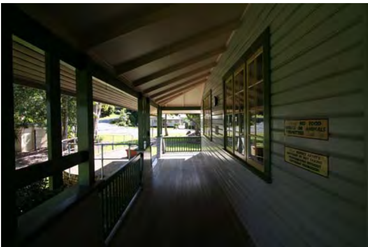
Photograph 21 Front verandah – modified but original fabric and Exceptional significance
