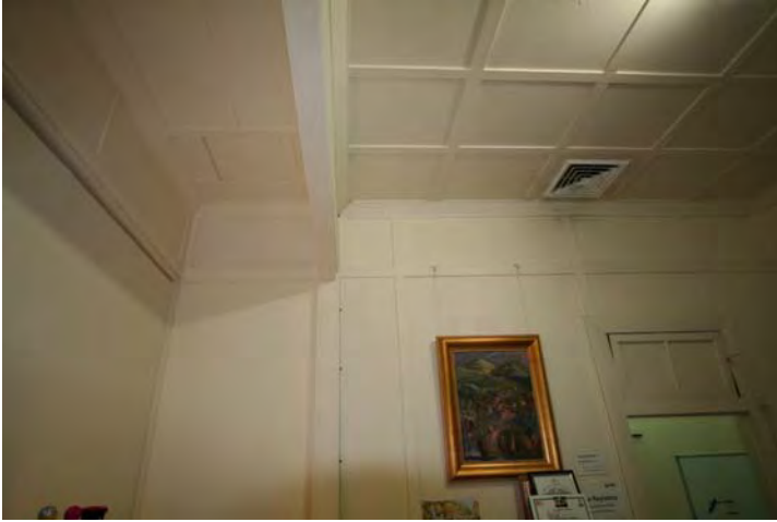
Photograph 106 Room layout altered and bulkhead remains
