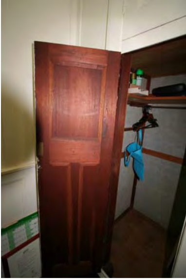
Photograph 126 Exceptional built in cupboard
