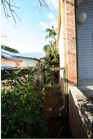
Photograph 43 The extension: Fabric and details – Moderate significance
