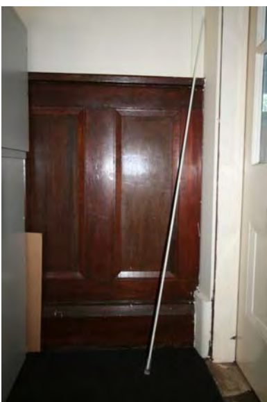
Photograph 84 Retained dado wall panel with original finish
