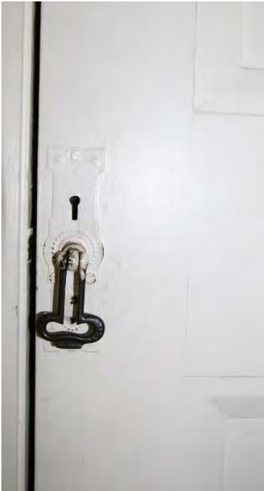
Photograph 113 Exceptional built in cupboard
