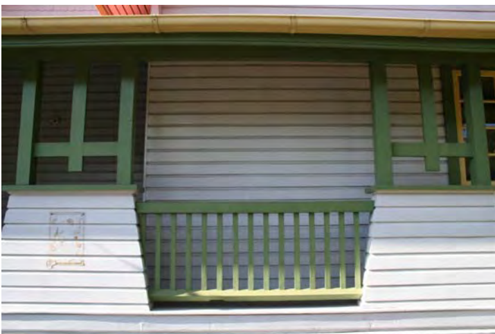
Photograph 39 Original fabric and details – Exceptional significance
