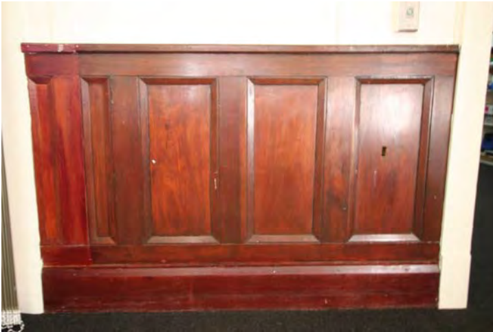
Photograph 85 Retained dado wall panel with original finish
