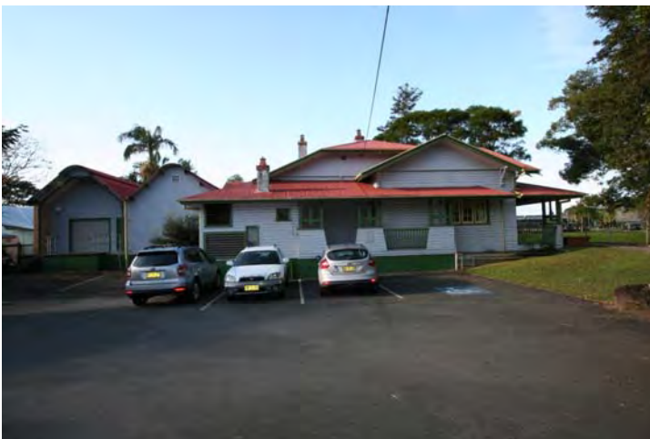
Photograph 66 The complete North Elevation and car park
