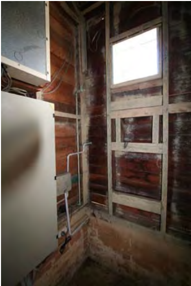
Photograph 14 Former laundry – modified and High significance
