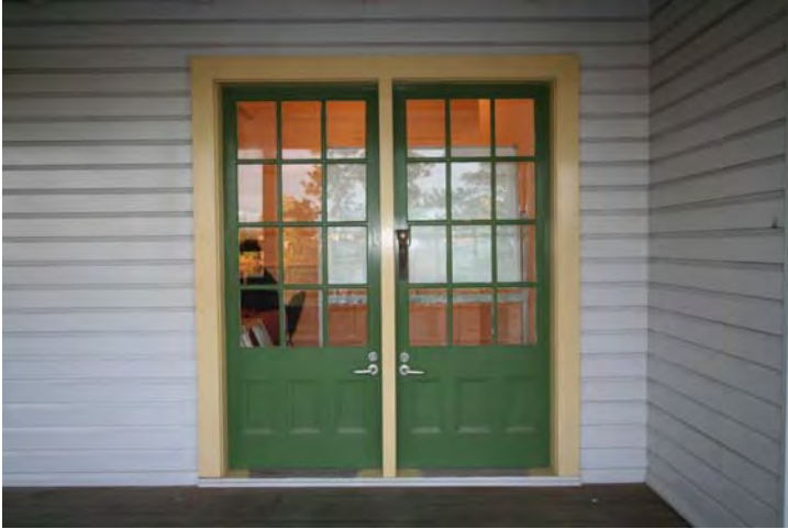
Photograph 70 Contemporary but sympathetic door set to verandah
