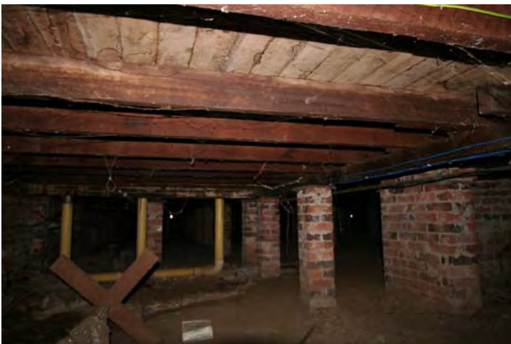
Photograph 9 Sub-floor view indicating generally sound conditions
