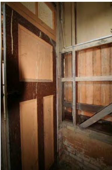
Photograph 12 Original store – former laundry – Exceptional significance
