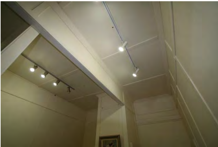
Photograph 115 Exceptional built in cupboard and removed wall with retained bulkhead
