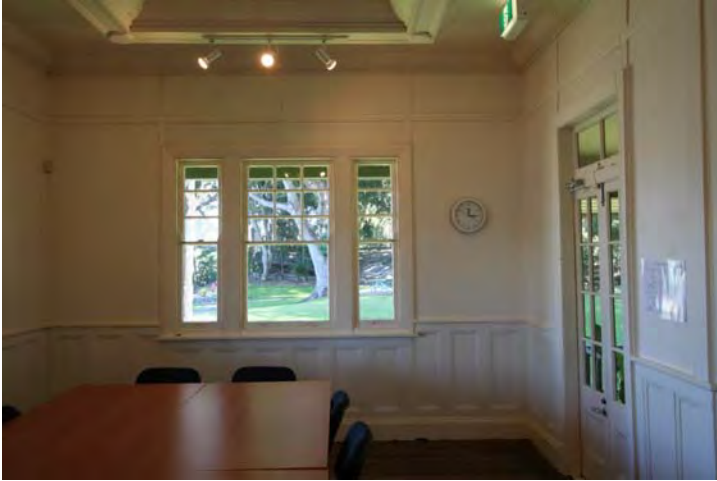
Photograph 4 Original windows and panelling – Exceptional significance
