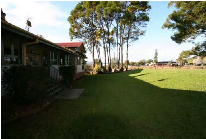
Photograph 59 Exceptionally significant front western verandah – lost front steps
