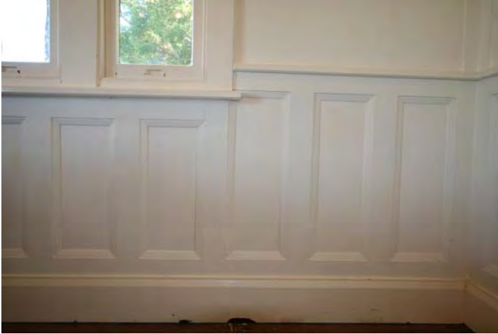
Photograph 149 Note paint removal from rare cedar joinery
