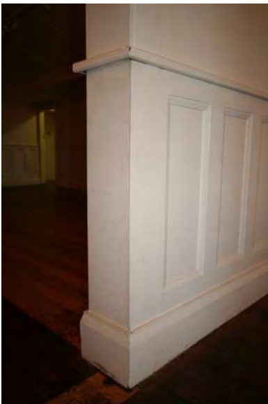
Photograph 145 Post enclosed in modified wall treatment
