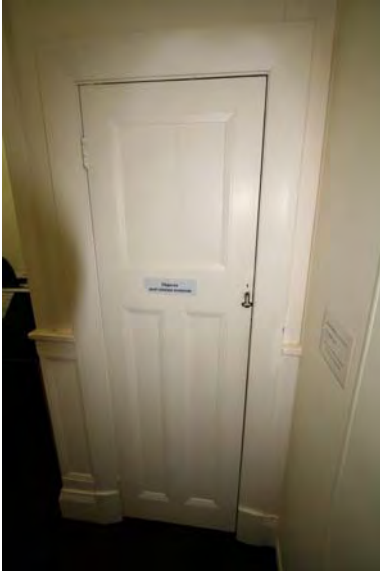
Photograph 112 Exceptional built in cupboard
