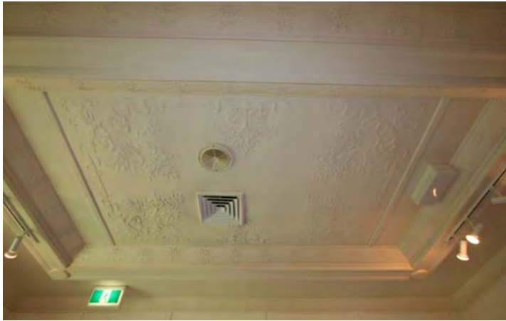
Photograph 1 The original ceiling – exceptional significance
