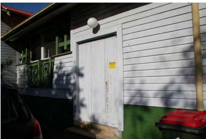
Photograph 24 Former laundry and verandah – Modified and Moderate significance
