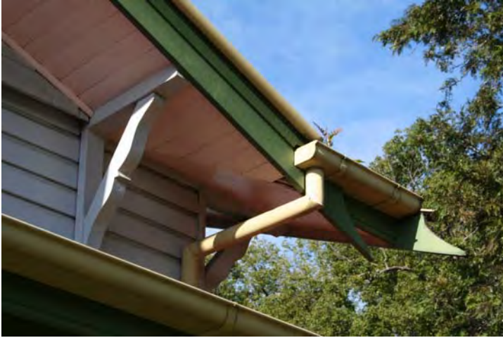
Photograph 37 Original fabric and details – Exceptional significance
