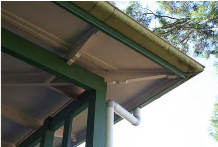
Photograph 32 Original fabric and details – exceptional significance (PVC Downpipes excepted)
