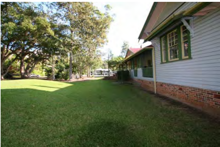
Photograph 60 Exceptionally significant front western verandah – lost front steps
