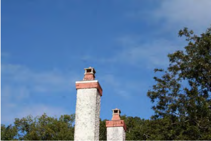
Photograph 40 Original fabric and details – Exceptional significance
