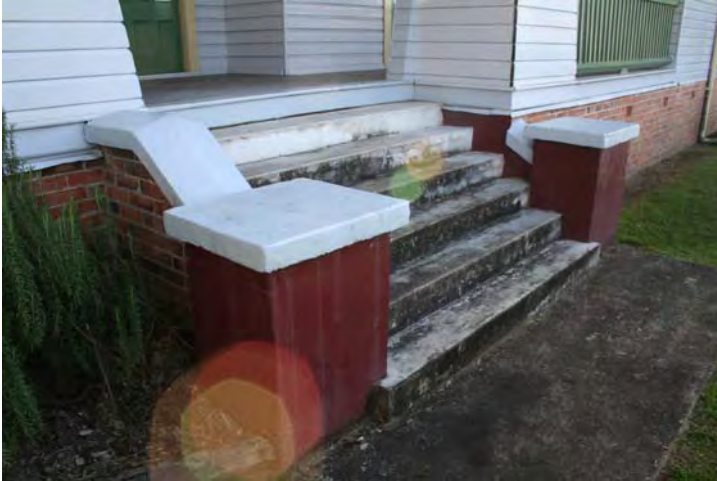
Photograph 31 Original fabric and details – exceptional significance
