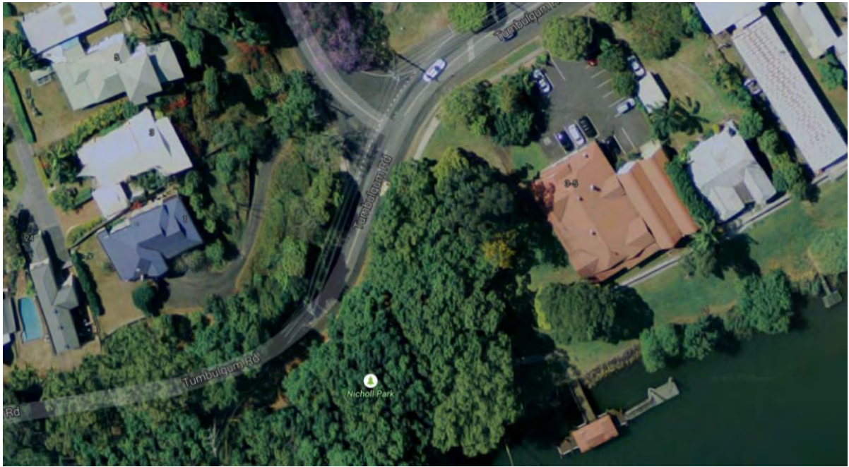
Figure 3 The former Proudfoot building is indicated by the tan coloured roofs and associated car park. Note the alignment of the northern remaining portion of Old Ferry Road with the concealed southern portion now within the Nicholl Park reserve and the symbolism of the current floating mooring.
