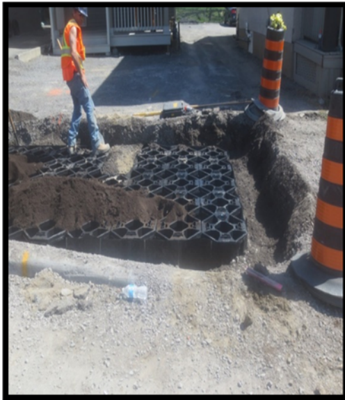
Statacell installation
