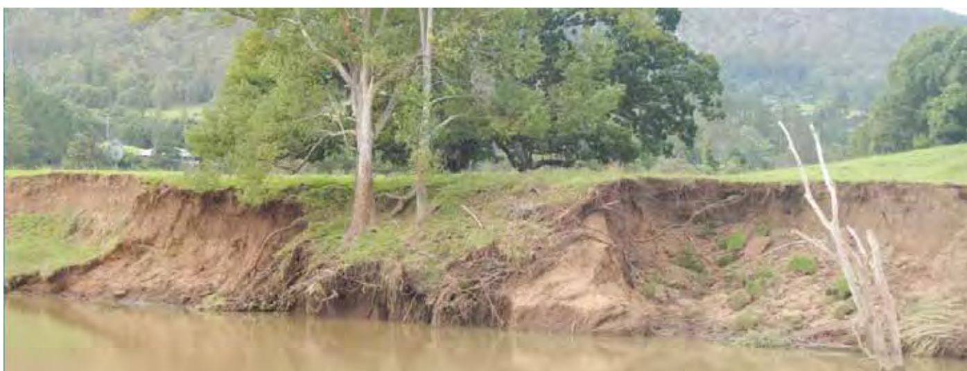
Waterway bank erosion on the Oxley River at Eungella. Photo Credit: Matt Bloor
