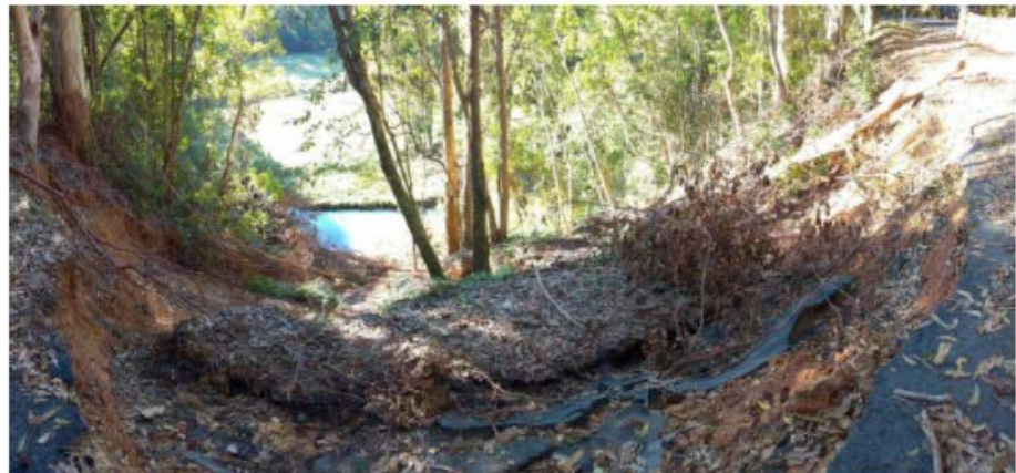
Photo 2: View looking downslope (east) from landslide back scarp
