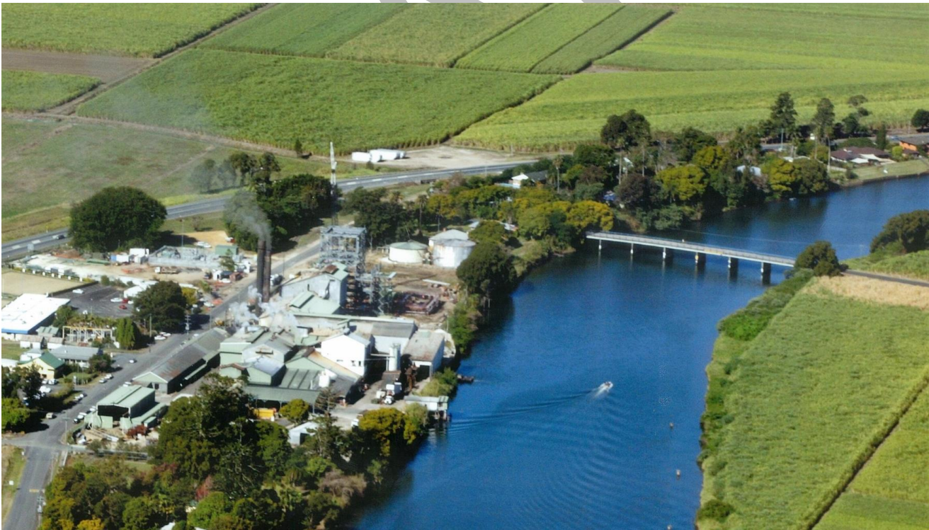
Figure 2 Condong Sugar Mill. Image courtesy of Sunshine Sugar
