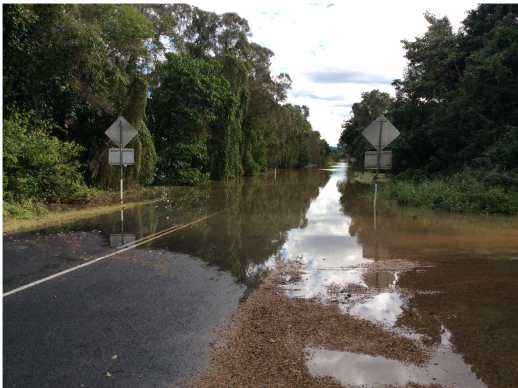
Photo 5 – Flooding impacts (June 2016)
