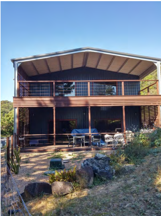
Figure 1 Unauthorised verandahs at rear
