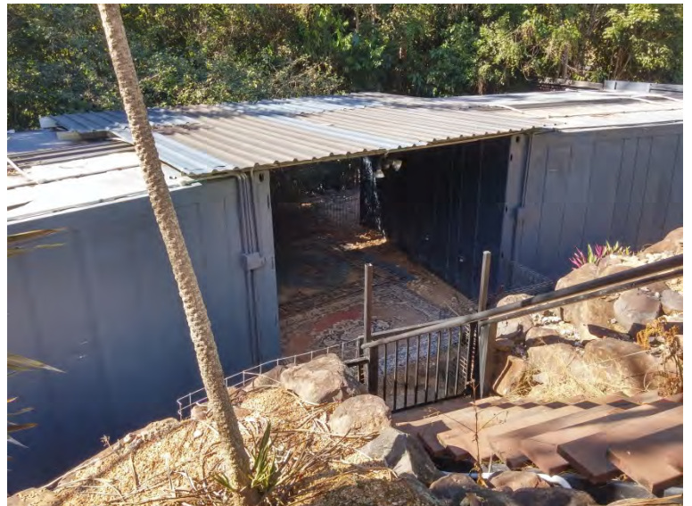
Figure 6 Four storage containers with awning
