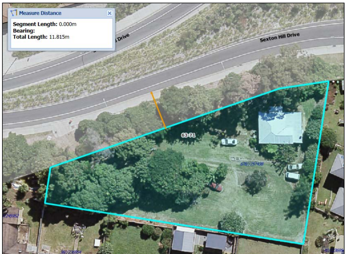
Figure illustrating the large setback between the property boundary and the road edge.
