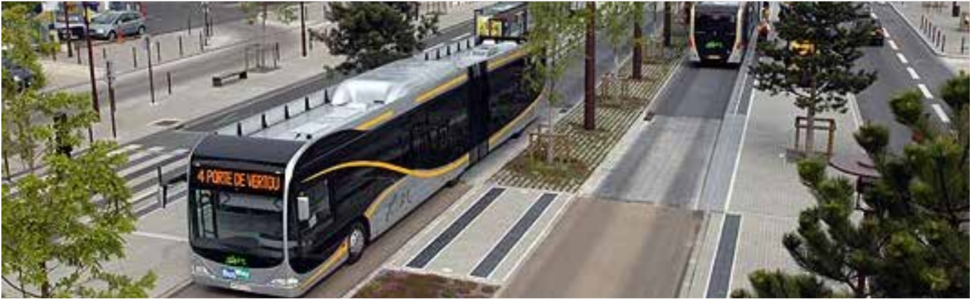
New Bus Interchange - The adopted Tweed Public Transport Strategy is to develop a Rapid Bus Transit Corridor Plan from Gold Coast Airport Transport Hub to Pottsville through Kingscliff with links to Murwillumbah.
