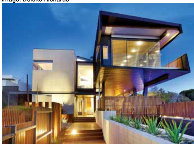
Principle 05 - Address the street - Provide a legible front entry with habitable rooms or decks which overlook the street. Image: Maddison Architects.
