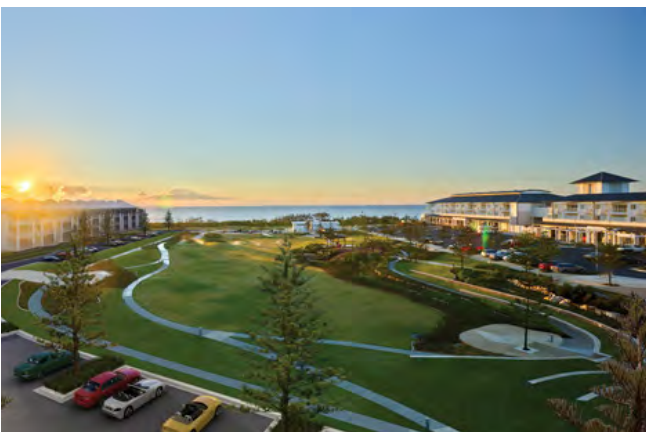
Salt Village Precinct accommodates two large tourism developments and small neighbourhood centre surrounded by predominantly low density residential characterised by large contemporary coastal homes.
