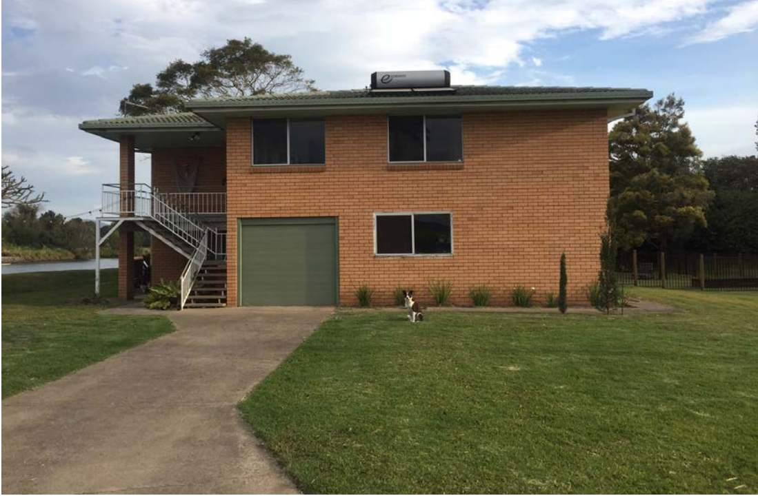
Figure 2: View of house from driveway
