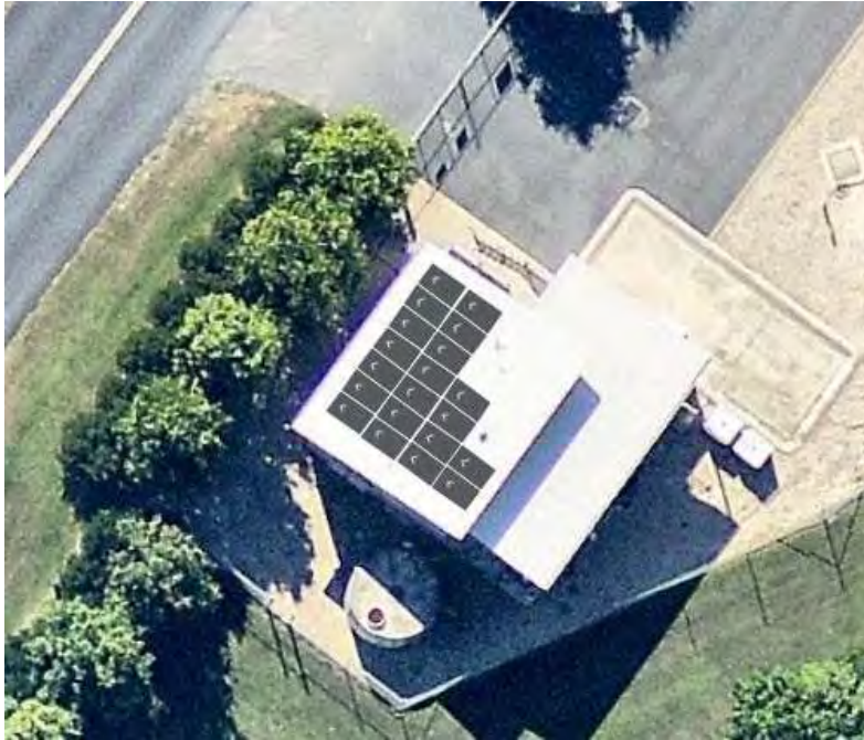
FIGURE 26: SOLAR PV ON MOOBALL WWTP 14
