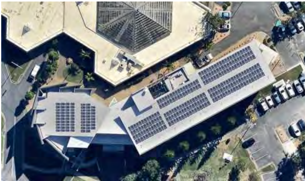
FIGURE 31: SOLAR PV ON TWEED HEADS ADMINISTRATION OFFICES 19
