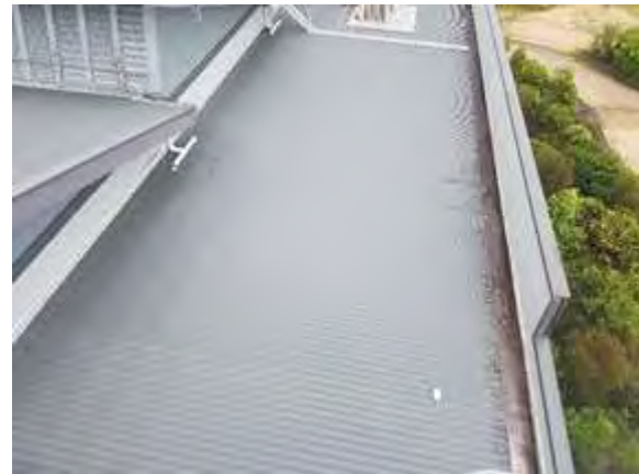
Flat roof to north
