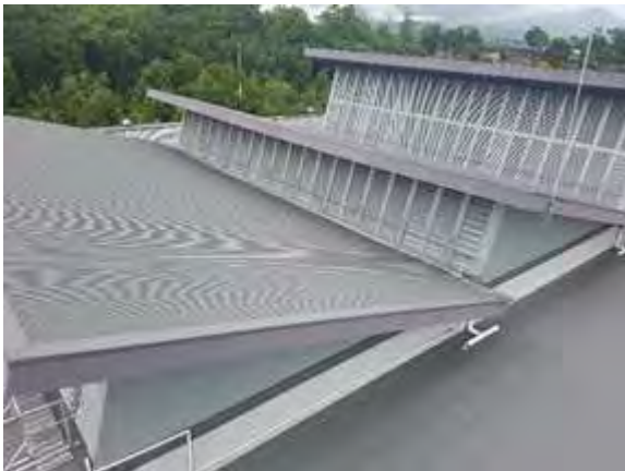
Western facing roof identifying setback for potential shading
