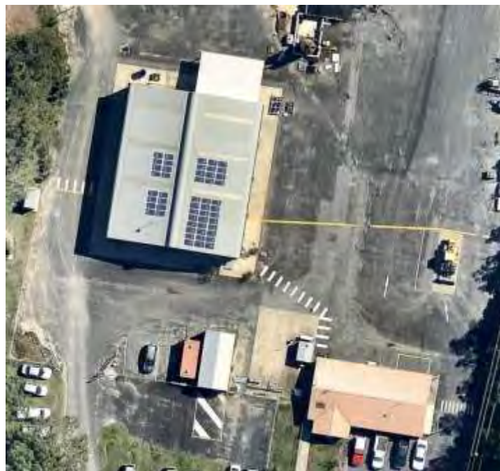
FIGURE 29: SOLAR PV ON TWEED HEADS DEPOT 17
