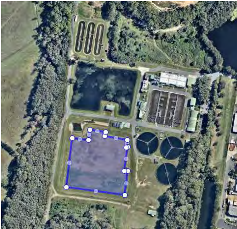
FIGURE 25: 700 kW SOLAR PV ON 14,370 m 2 LAND AREA AT BANORA POINT WWTP 13
