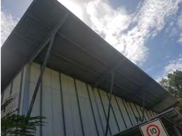
Roof structure looks suitable for install
