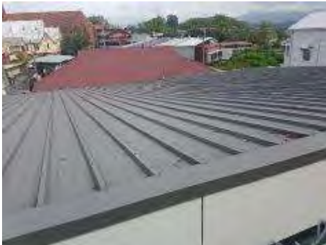
Proposed west facing roof for installation of modules
