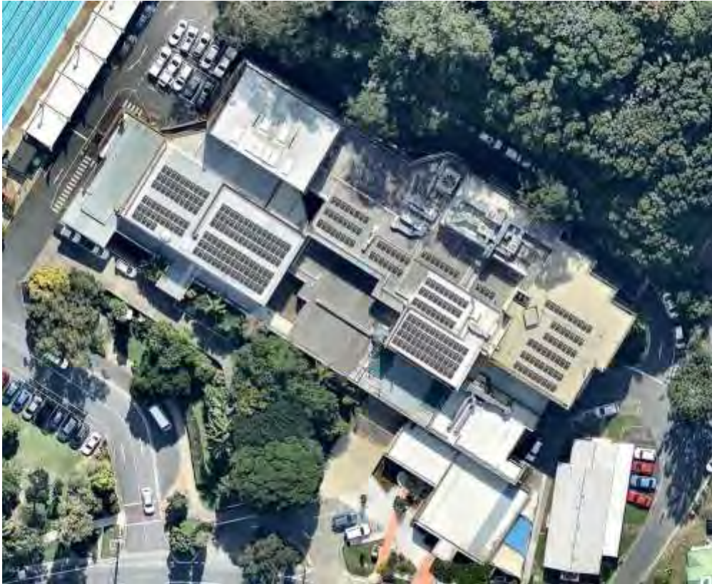
FIGURE 28: SOLAR PV ON CIVIC CENTRE BUILDING, MURWILLUMBAH 16
