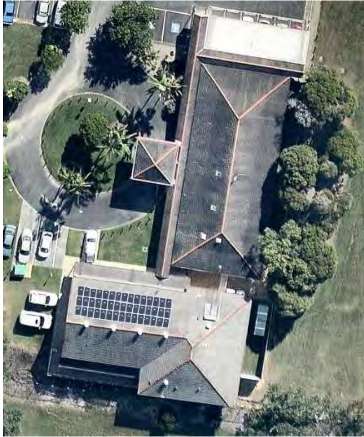
FIGURE 30: SOLAR PV ON SOUTH TWEED COMMUNITY HALL 18
