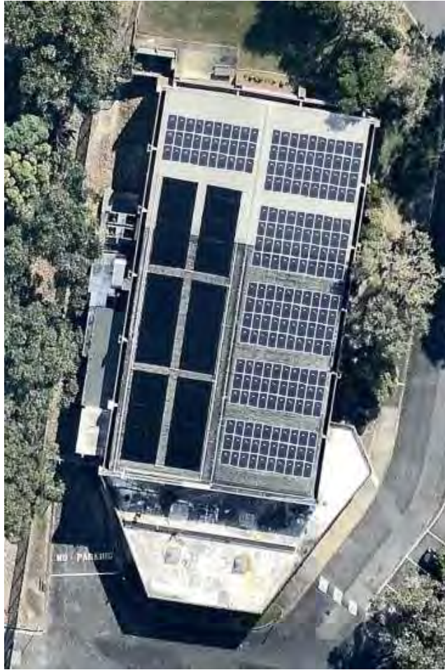
FIGURE 32: SOLAR PV ON TWEED HEADS SOUTH POOL 20
