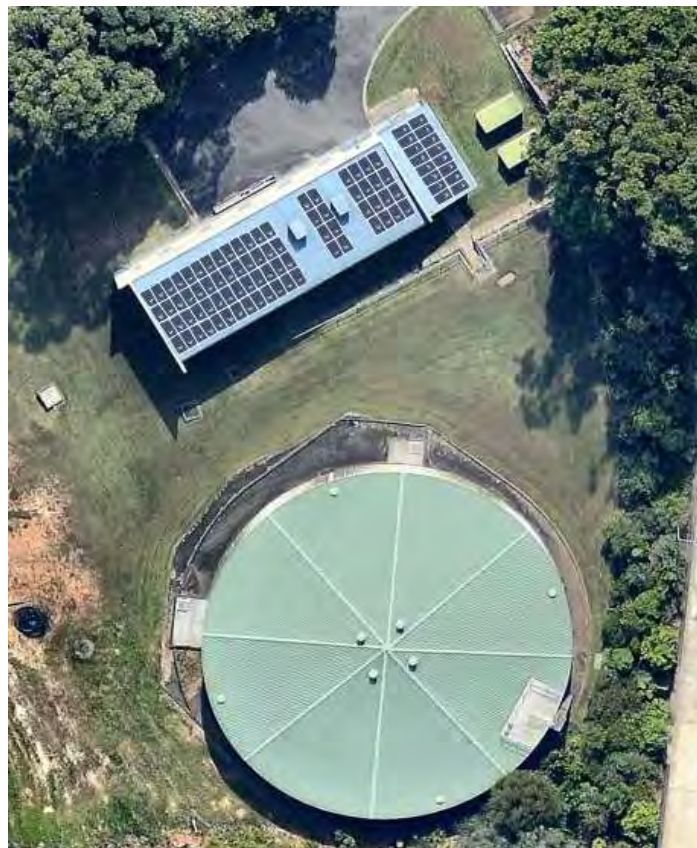
FIGURE 27: SOLAR PV ON BRAY PARK #2 WPS 15
