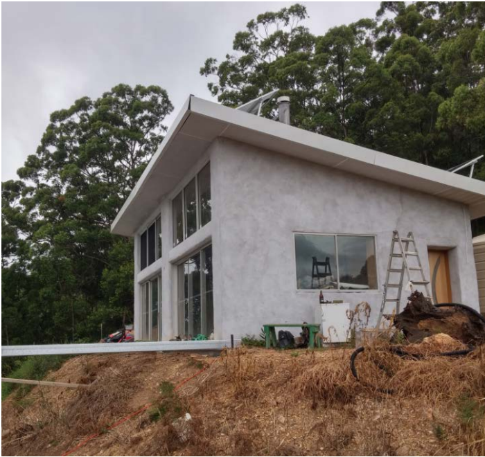
Side view of structure showing front door
