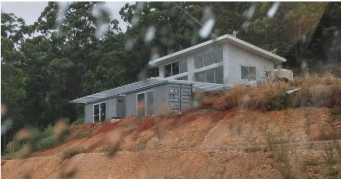
Structure with deck and two shipping containers
