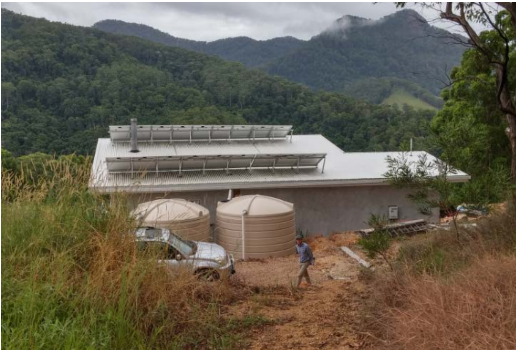
View from rear showing two rainwater tanks
