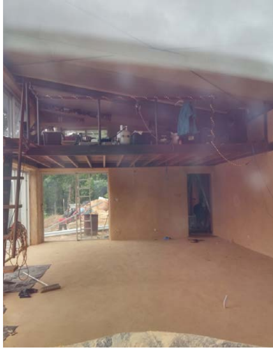
Internal view of structure showing mezzanine level and bathroom
