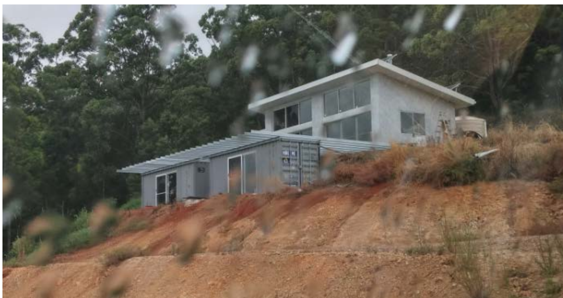
Structure with deck and two shipping containers
