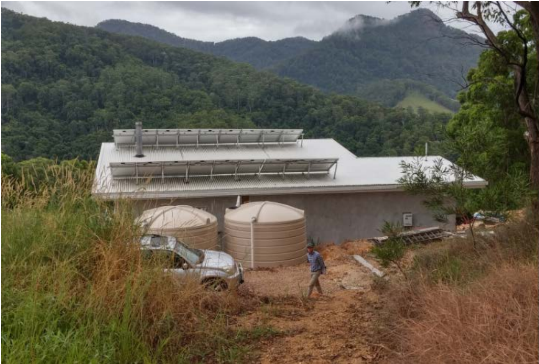
View from rear showing two rainwater tanks
