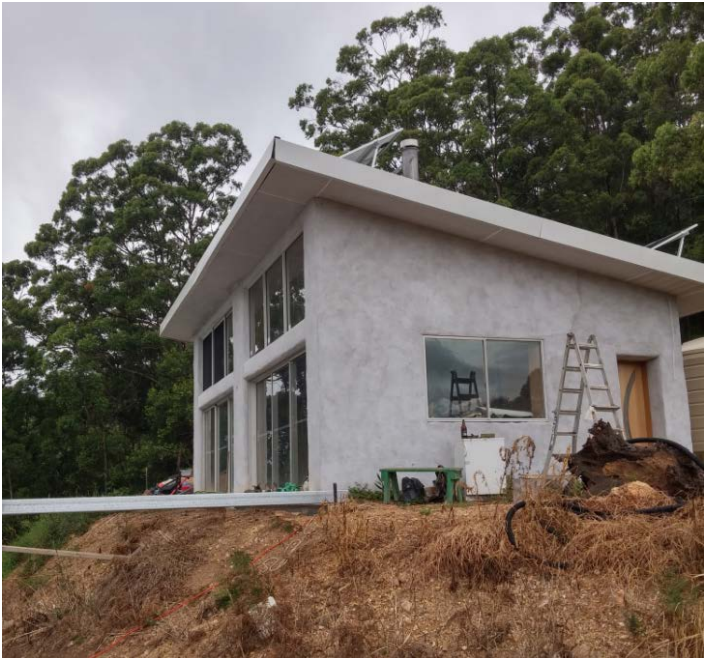
Side view of structure showing front door
