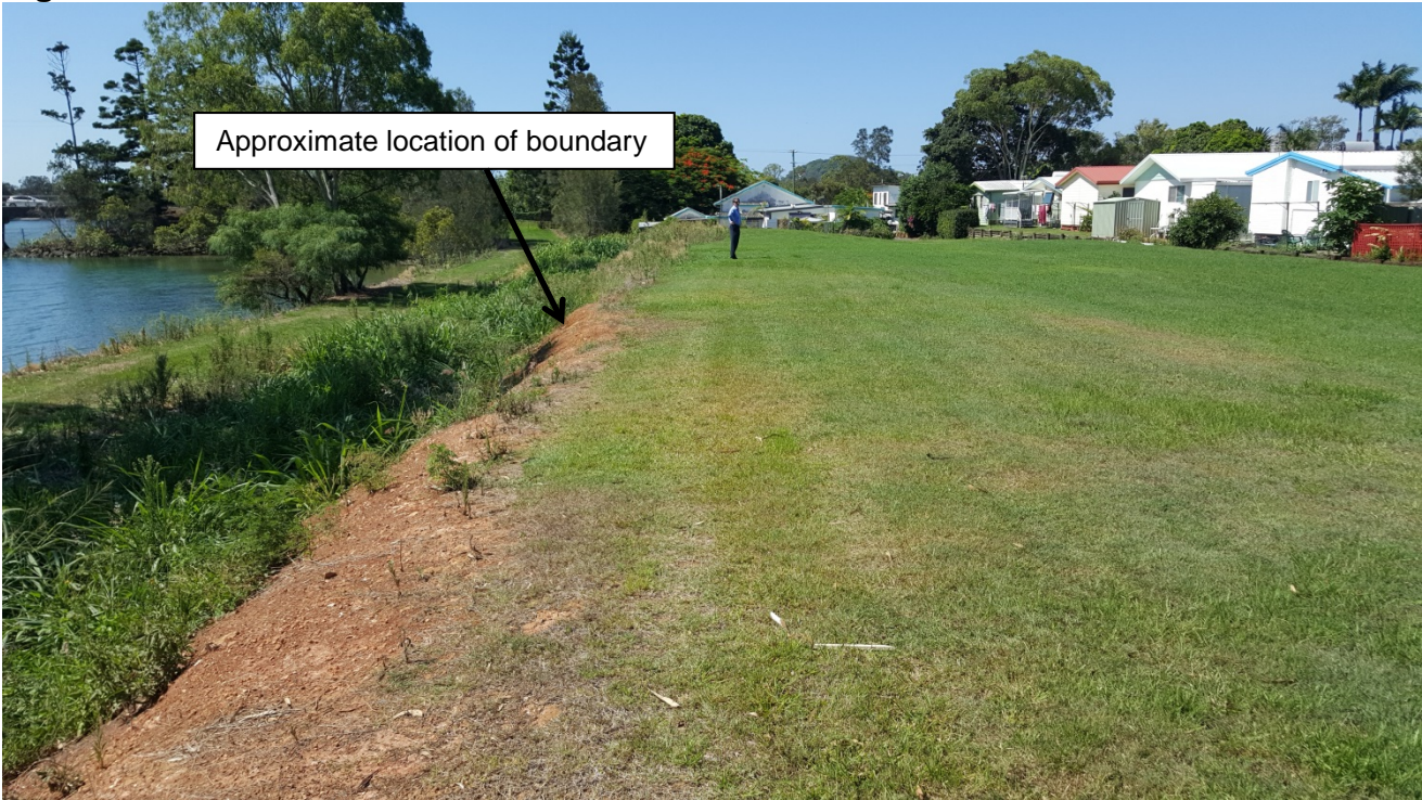
Figure 5: Extent of fill on the site.
