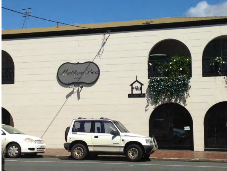
Figure 6: Unlawful Signage – January 2017
