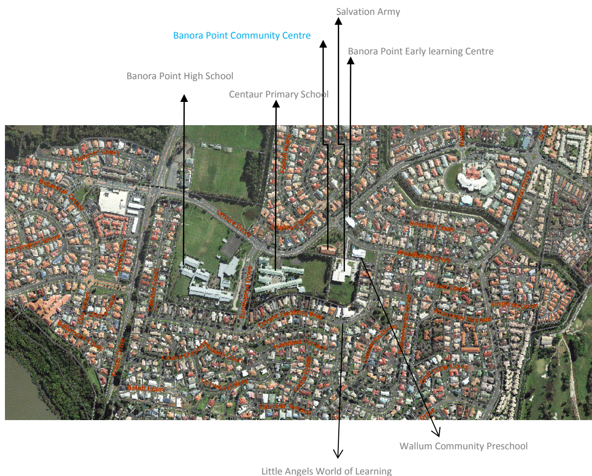
Figure 1. Banora Point Community Centre Location
