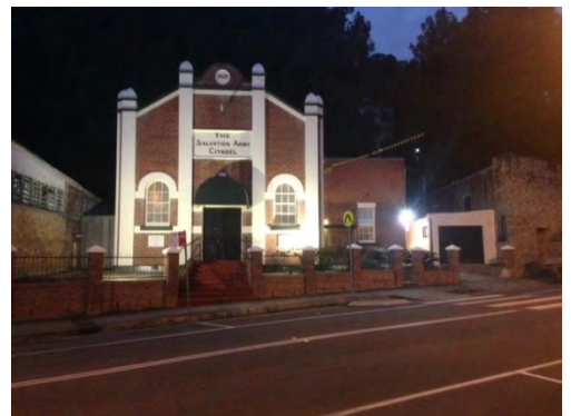
New exterior lighting (prior to front door installation)
