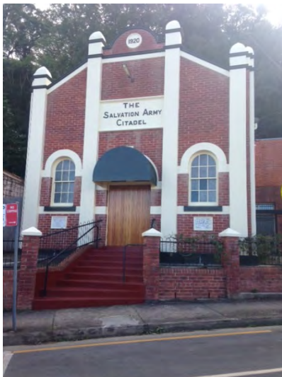
Street frontage and entry
