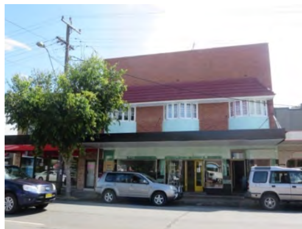
Wollumbin Street frontage after painting and pressure cleaning
