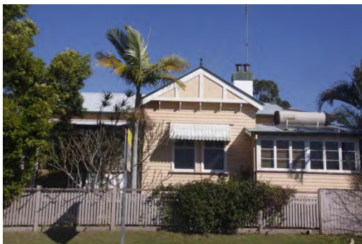
Side before (Prince Street)
