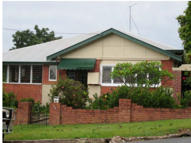
Front of house after with stucco painted in a neutral colour and new awnings and trims in colours appropriate to the period of the house
