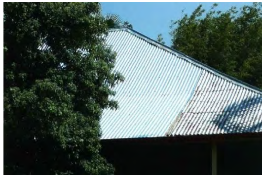
After replacement with galvanised sheeting
