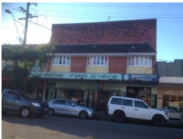
Wollumbin Street frontage before
