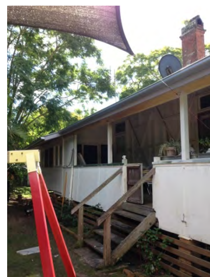
verandah guttering after
