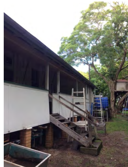
verandah guttering before
