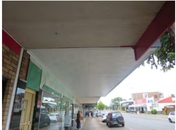
Awning cleaned, rust treated and painted
