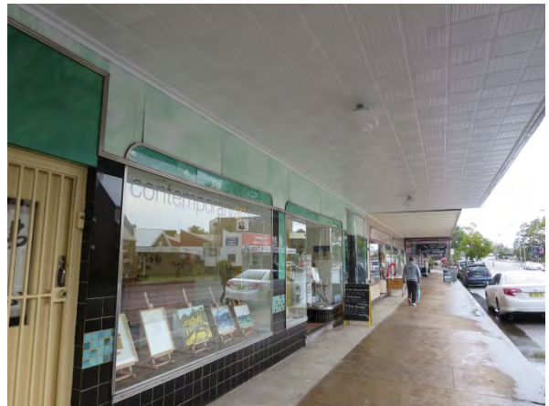
Awning cleaned, rust treated and painted and lighting installed
