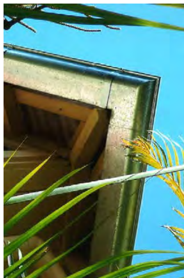
New galvanised guttering after
