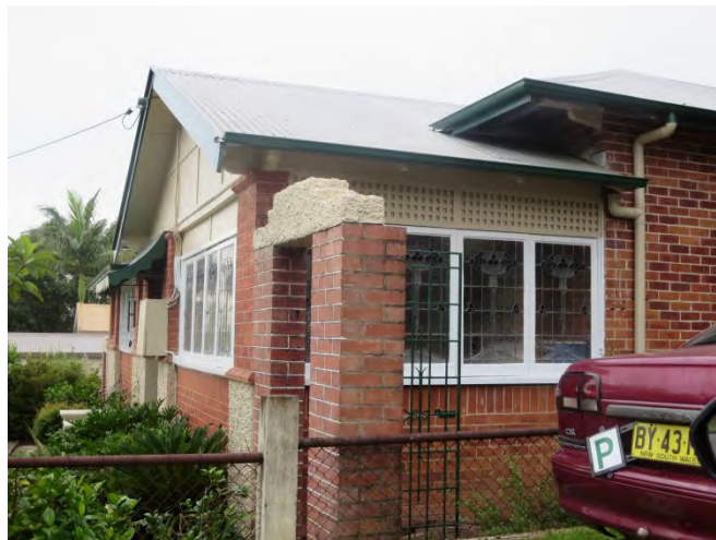
Side after with trims and windows painted
