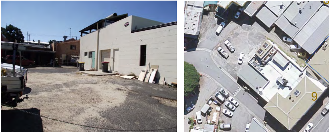
Figures 1 and 2: Photo & aerial imagery of rear car parking area
