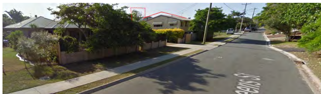
Figure 3: View of Site approaching from the south (Queen Street), the DA proposes to raise the existing dwelling on average 1.0m above that shown in this image and includes a roof deck some 2.02m above this (indicative works shown in red)
