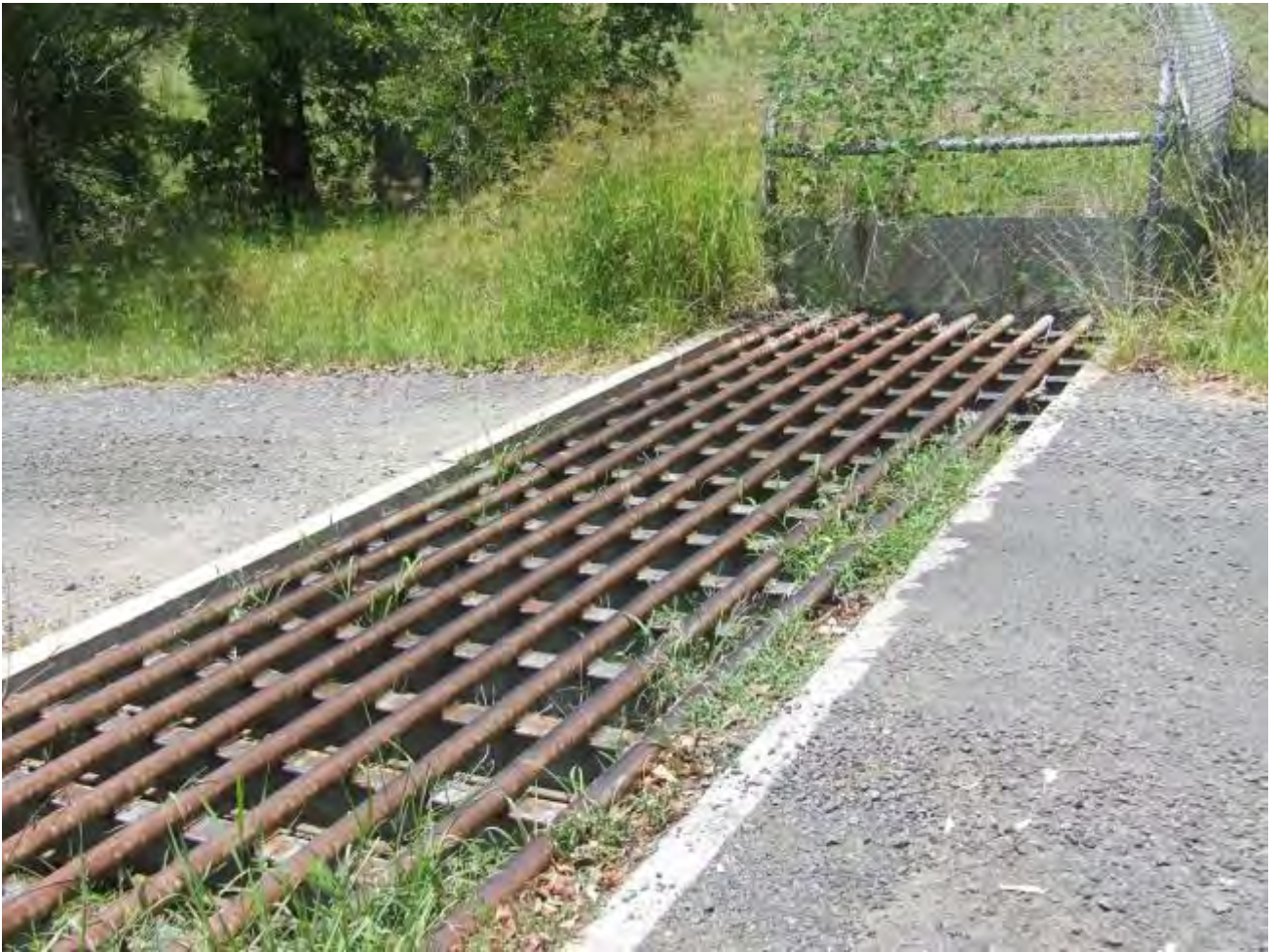
Figure 3 - Koala grid at rural driveway entrance
