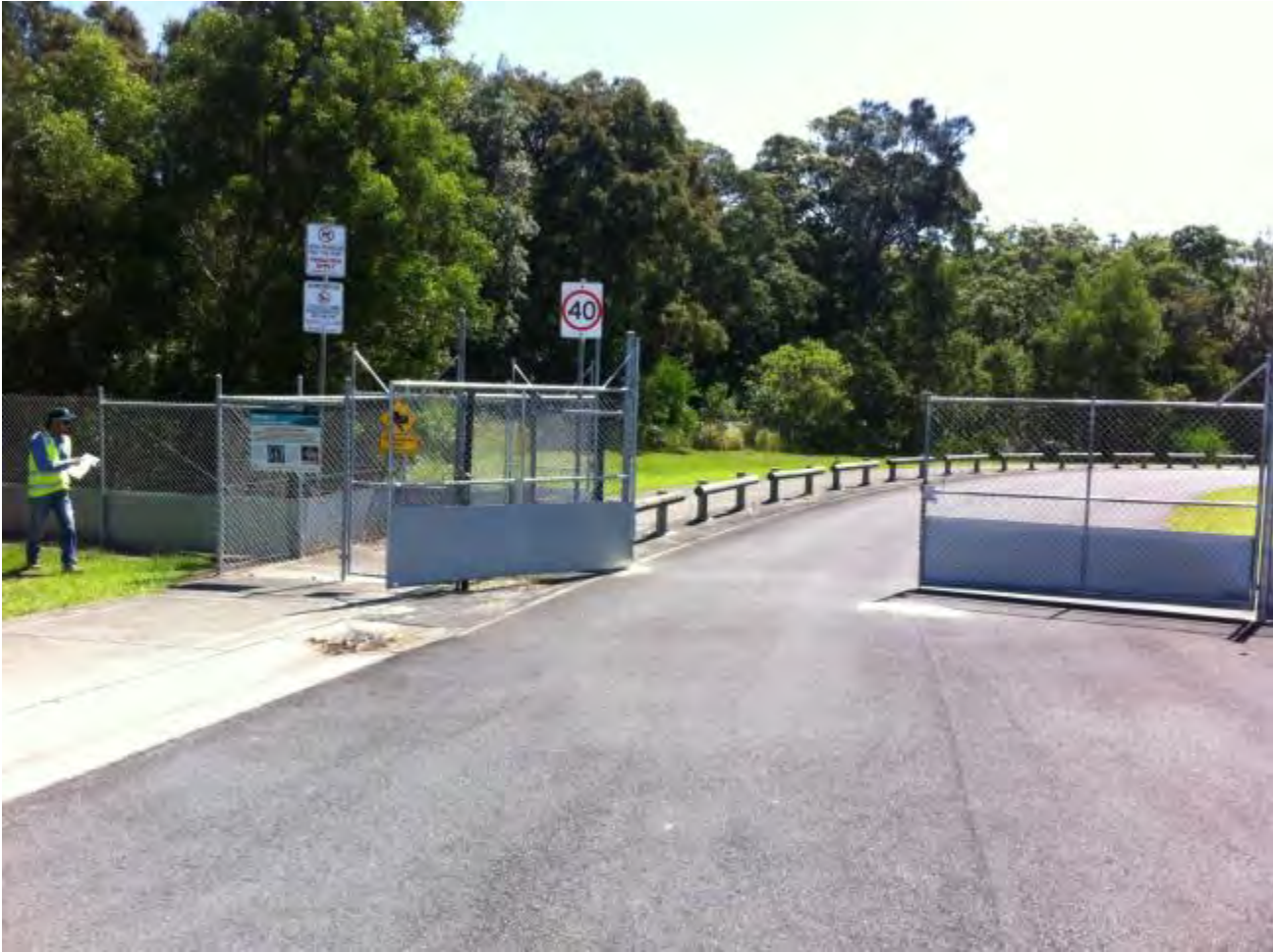
Figure 2 - Existing vehicle entrance gate with pedestrian access to the left
