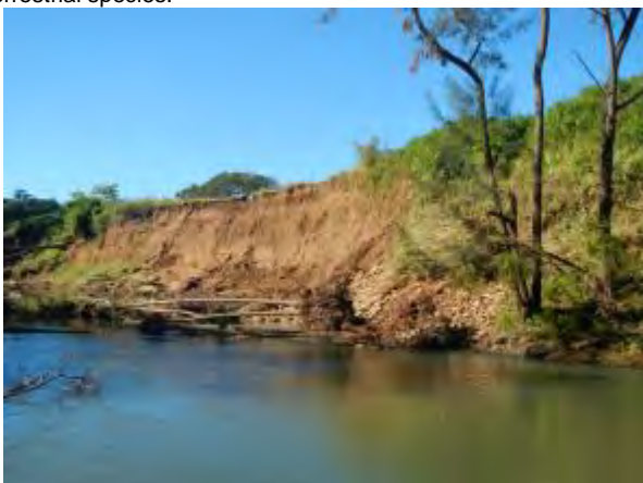
Bank erosion, Oxley River. Significant planning during the first quarter has been required prior to rehabilitation in second and third quarters 2016.
