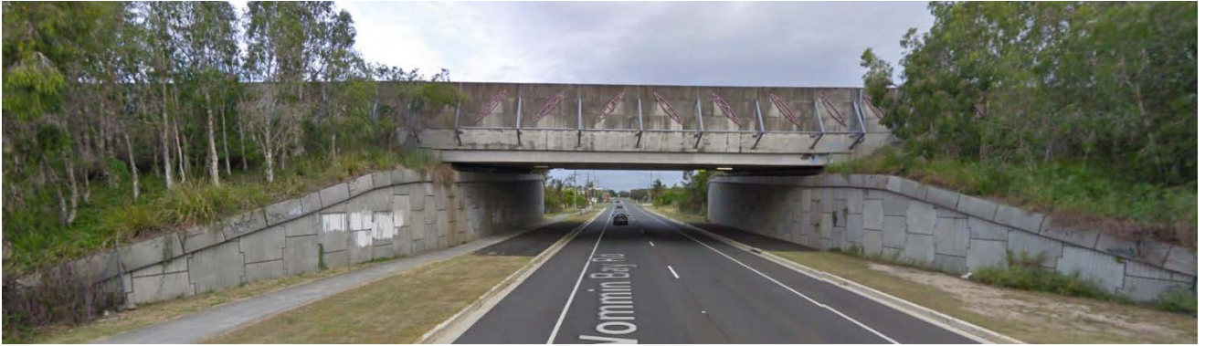
Wommin Bay Road at the Pacific Highway underpass (eastbound)
