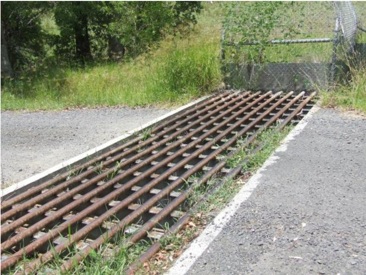
Figure 3 - Koala grid at rural driveway entrance
