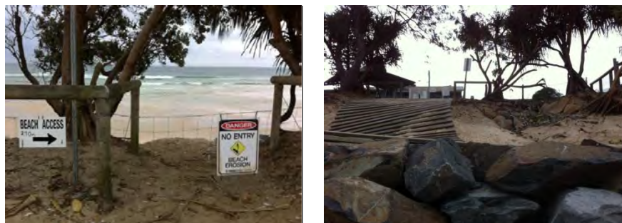
Figure 3-1 Example of Closure of Unsafe Beach Access by Council Following Erosion
