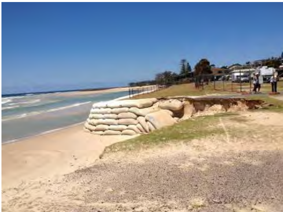
Figure 3-3 End Effects at Geotextile Sand Container Wall at Kingscliff Beach Holiday Park (from NSW Government, 2011)
