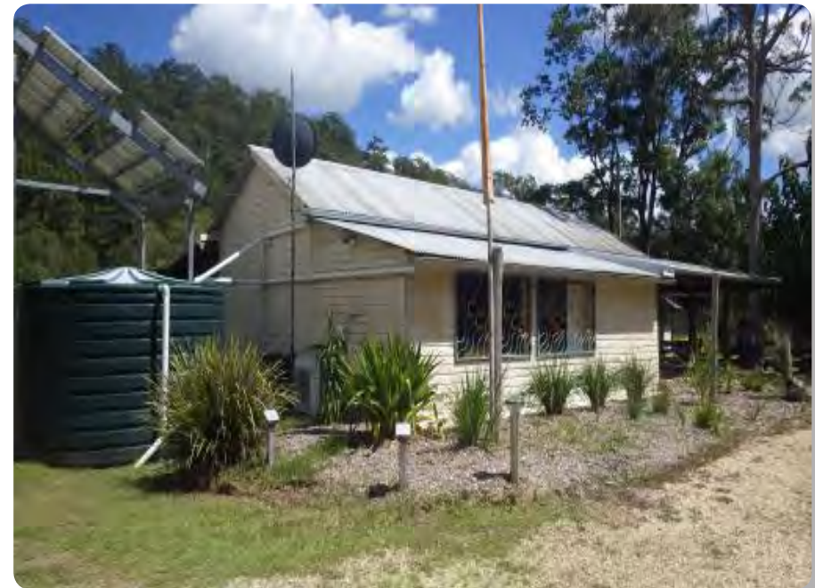
Chillingham Community Centre
