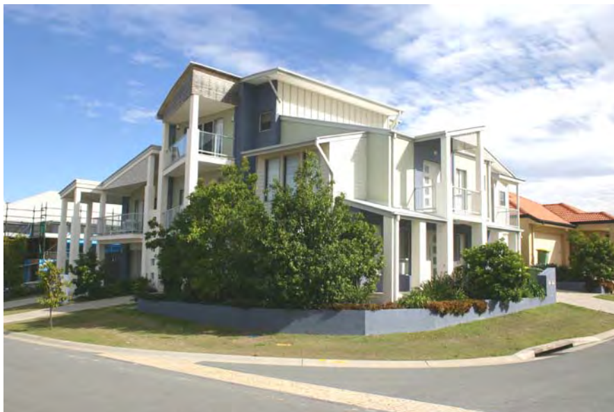
This building addresses its corner location by designing both street elevations with equal importance.
