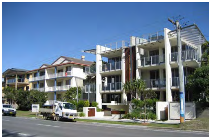
These residential flat buildings all have their primary orientation to the street with external living areas, low height fences, entries, windows and doors.
