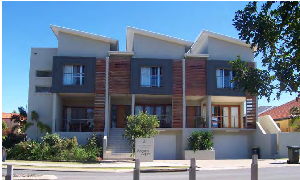
The impact of ramps and garage doors to this basement carpark has been reduced by making the garage doors in line with the buildings elevation and making the doors solid so as to read as the base and wall of the building, Ideally it would only have one entry.
