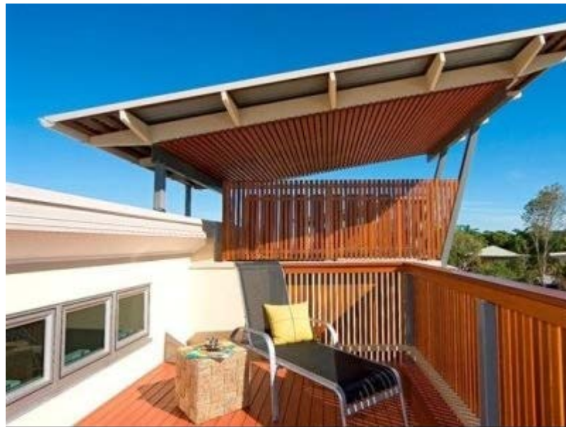
Figure 1: Successful roof top deck (stepped into the top storey, consistent materials and partially roofed for useability)
