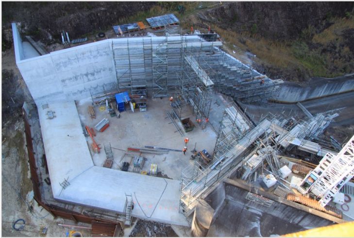
Clarrie Hall Dam Spillway Upgrade
